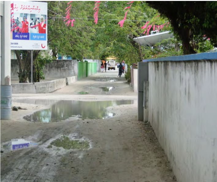
Water collected at junction. Closed by playground.
