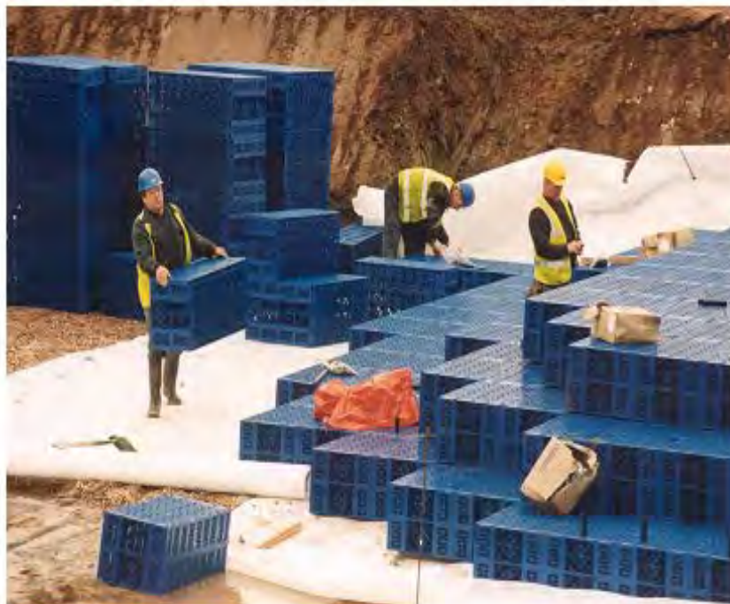
Figure No. 6.5: Proposed underground tank for the storm water storage
