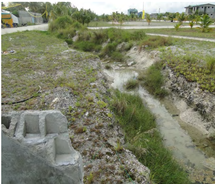
Earthen drain constructed by council
