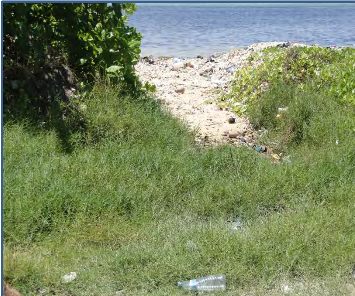
Existing out fall to be regularize by constructing pipe culvert cum flap gate
