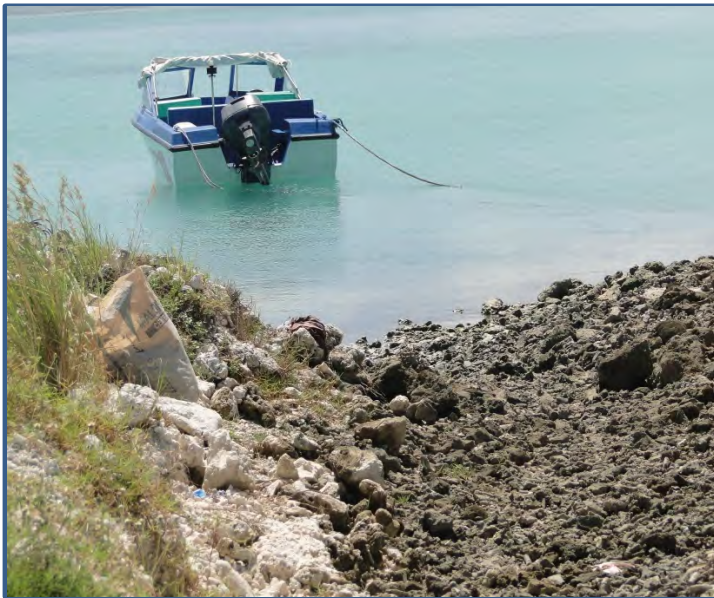
Existing out fall to be rehabilitated after constructing culvert cum flap gate
