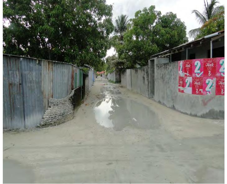
Link road to be filled to match the slope towards as main drainage path along the main road
