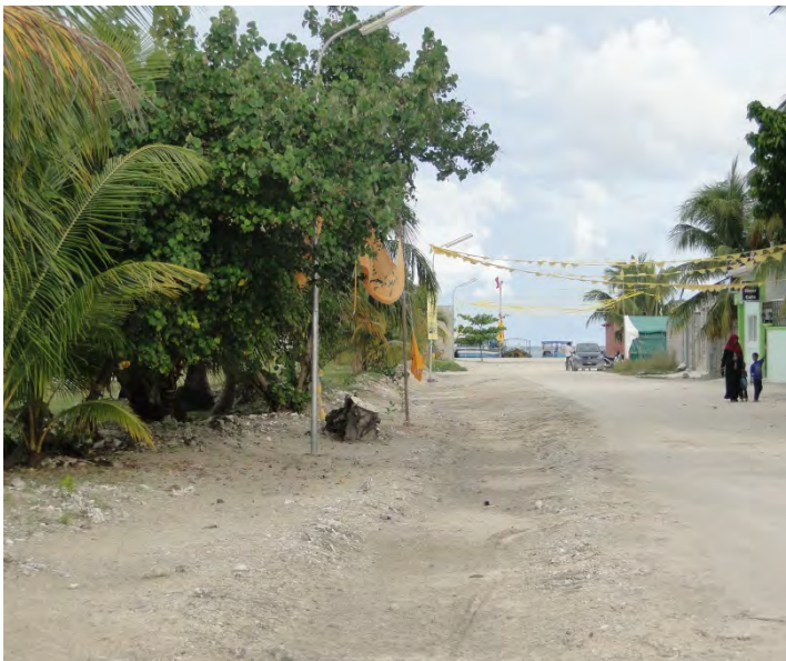
Earthen drain along the road – constructed by council
