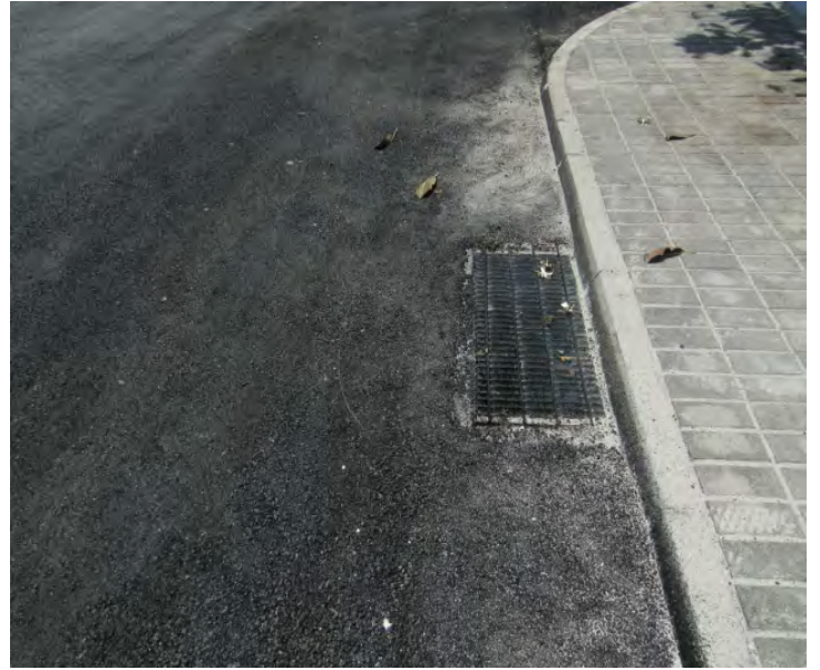
Newly constructed asphalt road with gully grating
