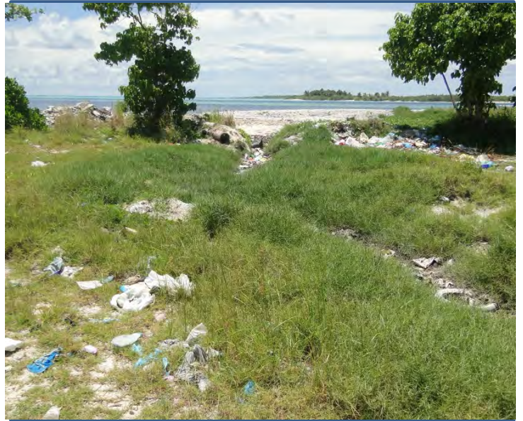
Existing outfall to be regularize by constructing pipe culvert cum flap gate
