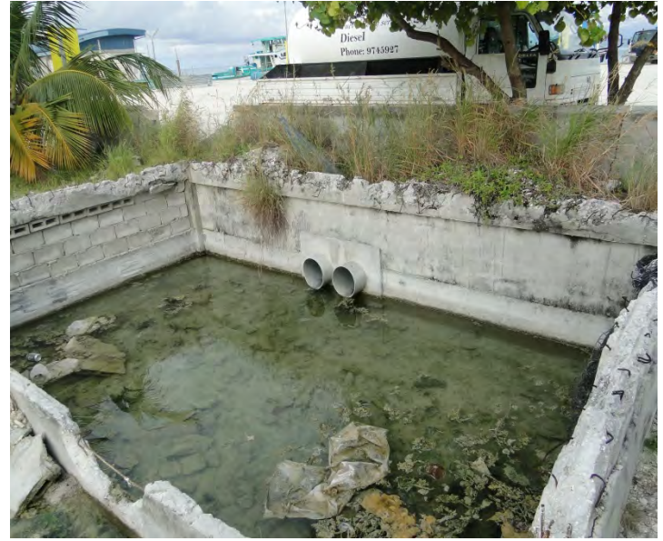
Existing drainage inlet – upstream of the sea
