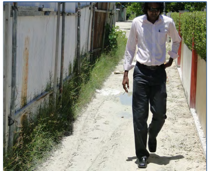
Flooding area without proper outfall
