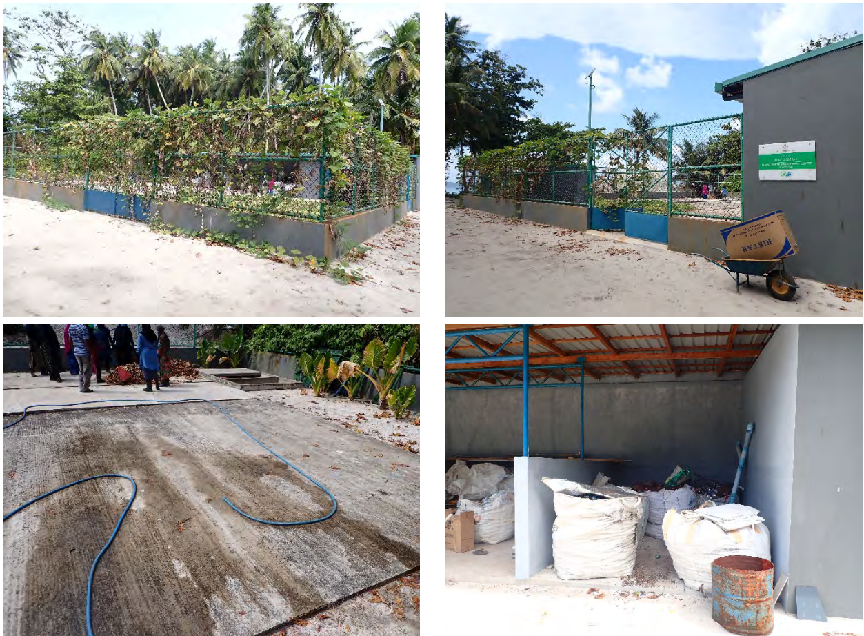
Figure 3. Images of the waste management site at present
