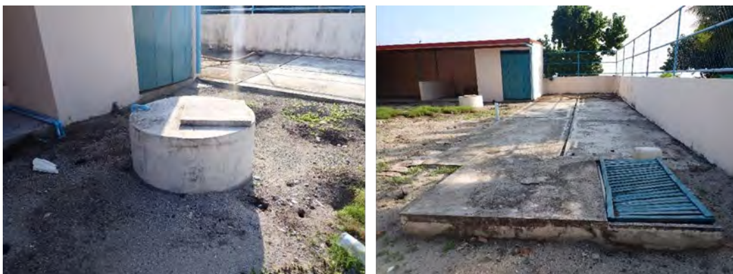
Figure 8. Existing groundwater well (left) and compost slab (right)
