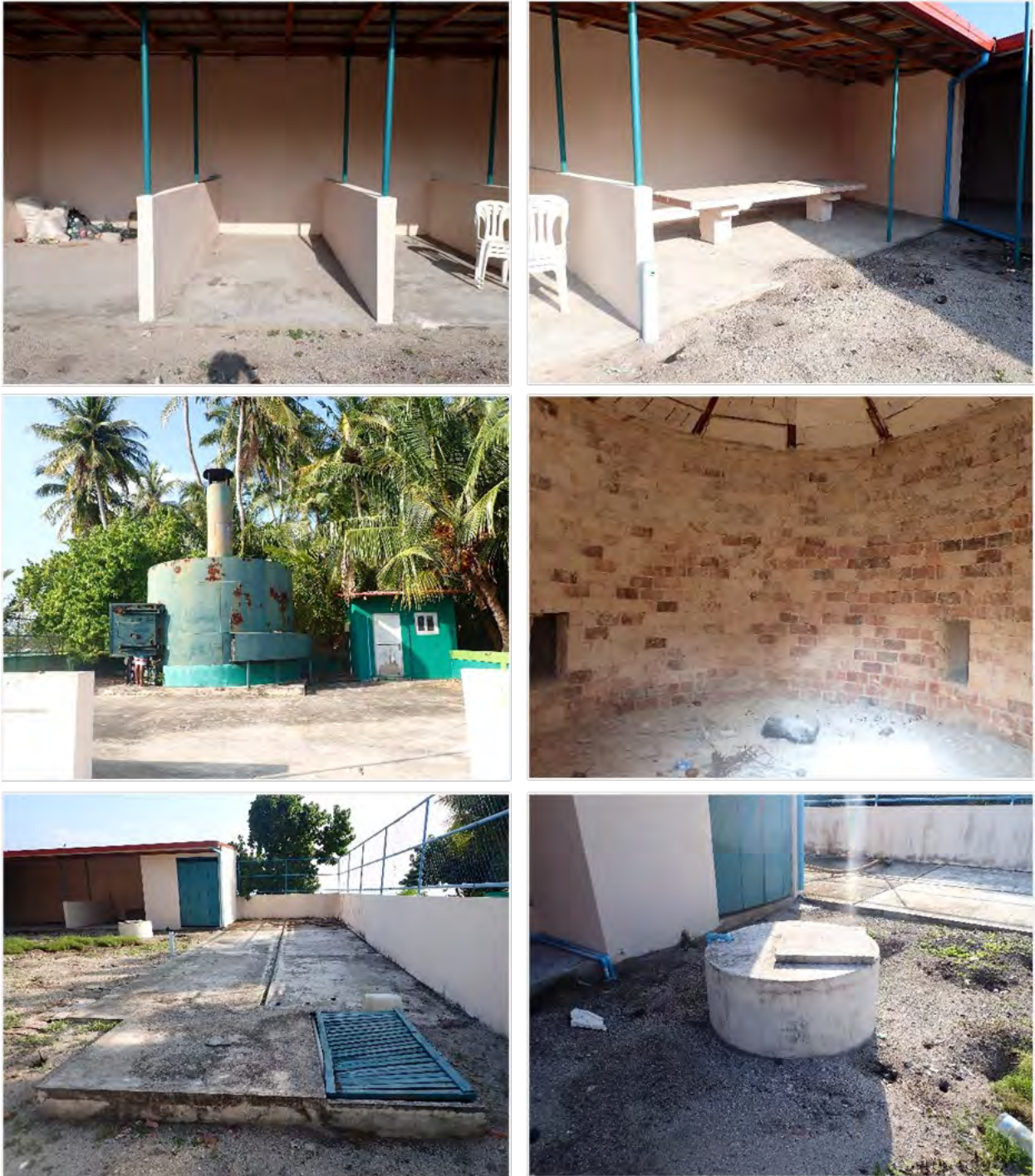
Figure 3. Images of the waste management site at present
