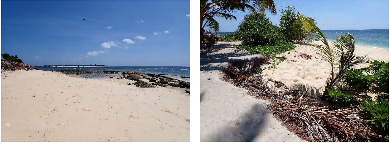
Figure 10. Beach adjacent to the IWRMC where erosion is being experienced
