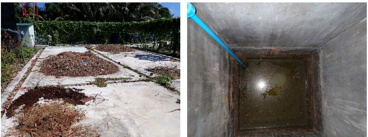
Figure 8. Existing compost slab (left) and groundwater well (right)
