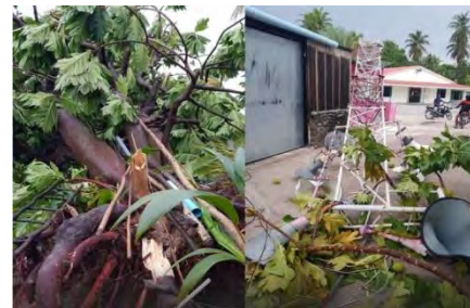
Figure 15 Trees uprooted due to wind damage in R. Vaadhoo. Source: Mihaaru
