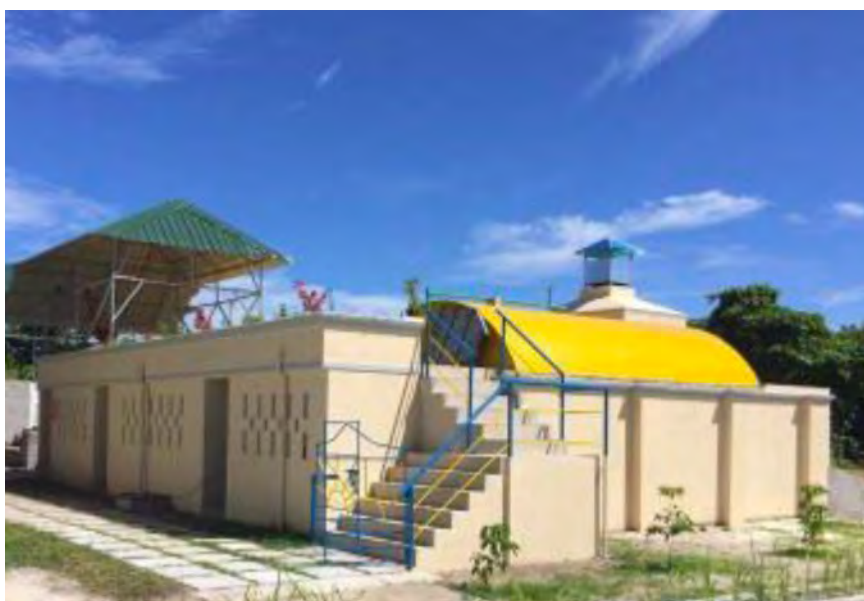
Figure 5. Example of AD plant installed in a resort hotel, Reethifaru, Baa atoll (source: BIOGEN, India)
