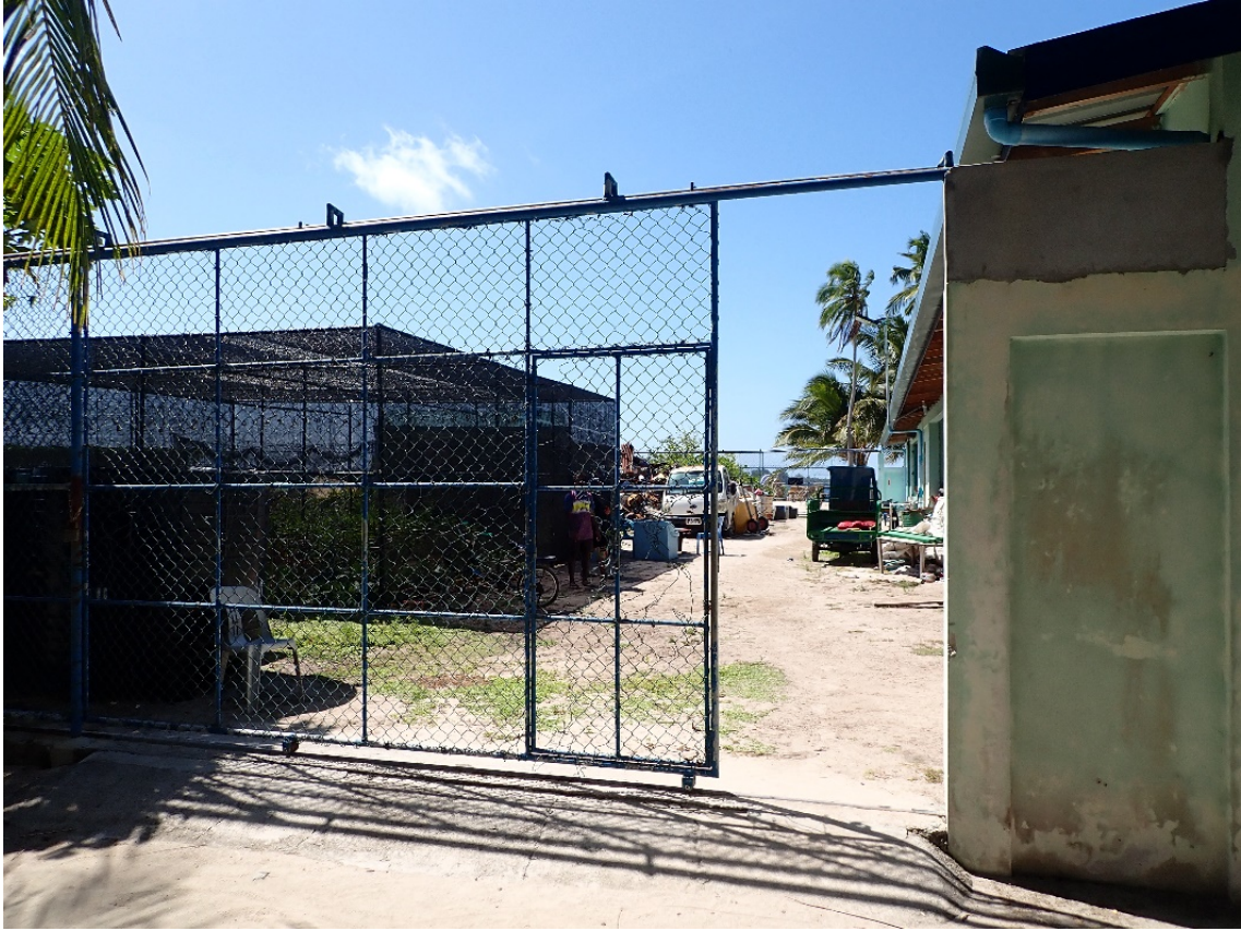
Figure 2. Images of the waste management site at present
