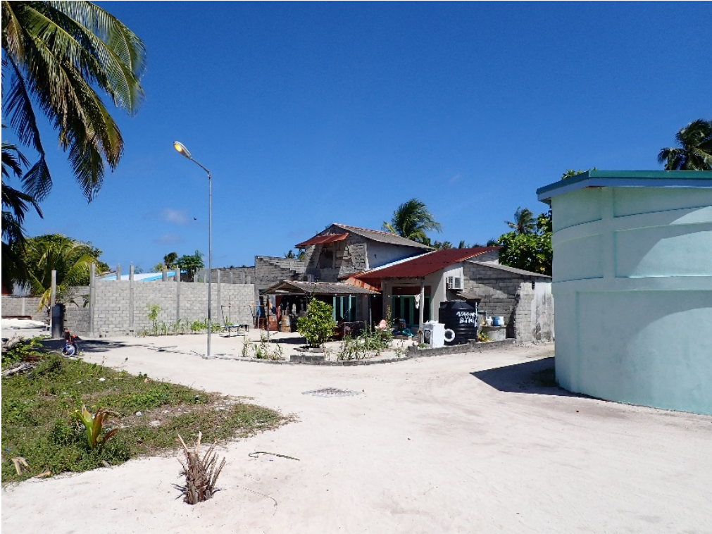
Figure 11. Construction site adjacent to IWRMC site
