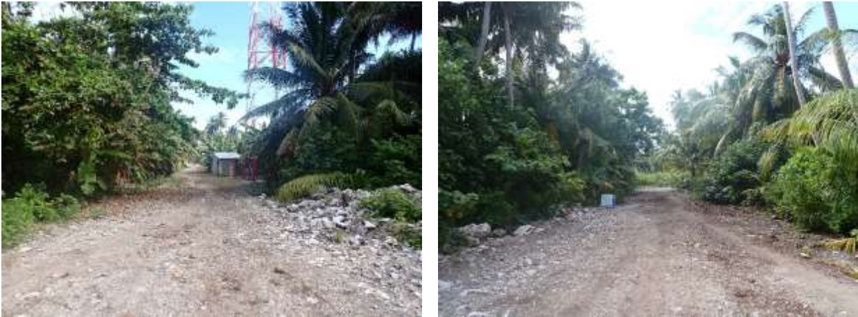
Figure 7. Road connecting IWRMC to harbour front road
