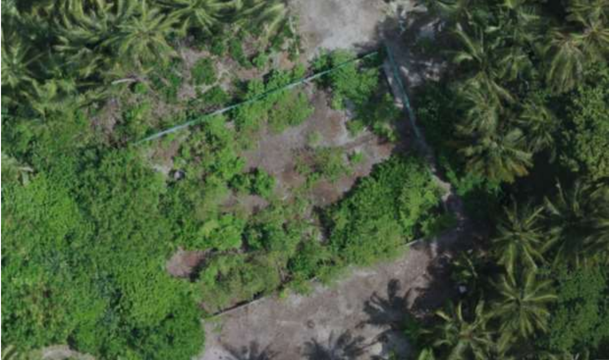
Figure 6. Drone image of IWRMC at Vandhoo. The boundary wall and some of the civil works are completed at the time of field visit
