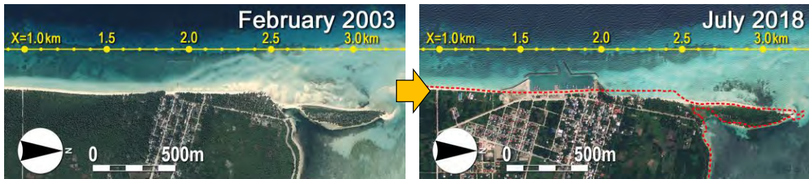
(1) Coastal Erosion due to Harbor Construction (Gan in Laamu Atoll)
