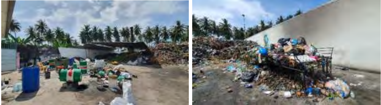
Figure 10. Ground of IWRMC is contaminated with waste oil and leachate from waste.
