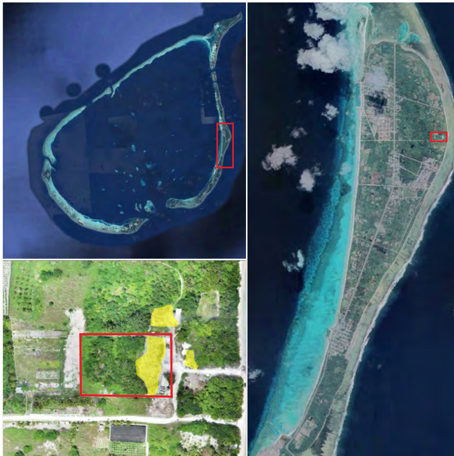
Figure 1. Location of Gan in Laamu Atoll (left top), proposed location of IWRMC (right, red highlight) and closeup of IWRMC (left bottom) with current waste disposal areas (yellow highlight)
