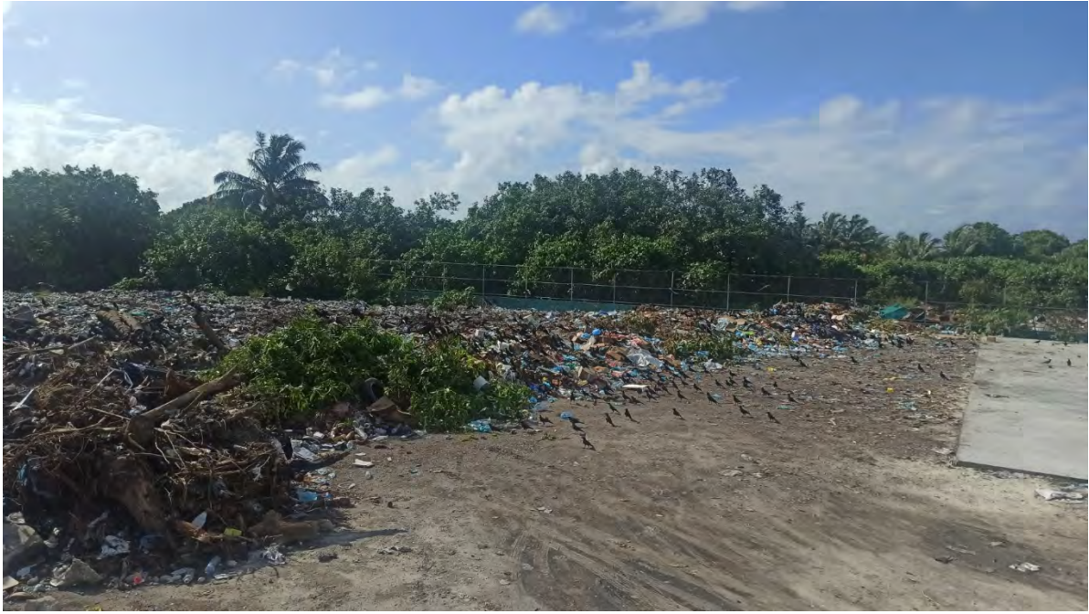
Figure 19. IWRMC site after recent vegetation clearance work undertaken by the Council (March 2021) – photo taken from SE corner looking towards NW side of plot (photo by L. Gan Island Council)
