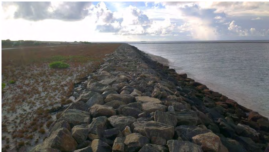
Plate 3: rock revetment on Khuldhufushi (taken in October 2012 J Hills)
