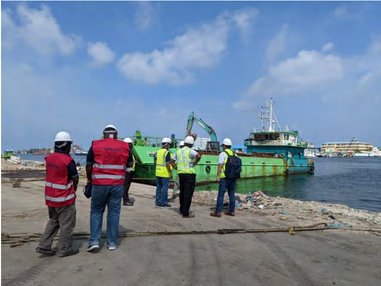
Inspecting ship ramp
