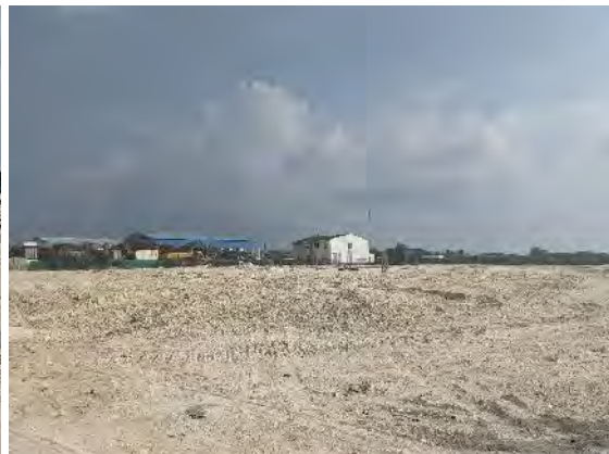
Filling and grading works (to reach +3.0 on top of slab)
