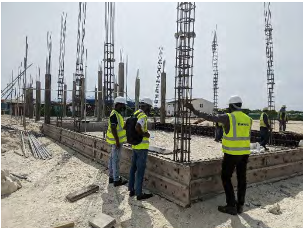
Admin Building foundation beam work
