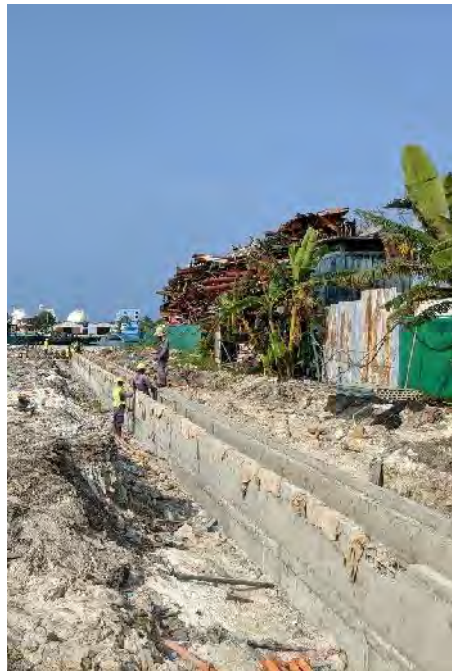
Trench-H (works on going)
