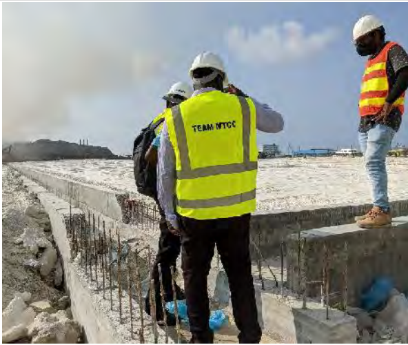
Trench-B,C intersection (revising the last piece a bit)
