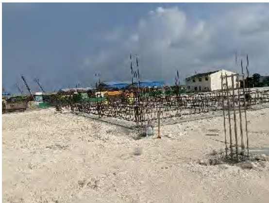
Admin Building foundation beam work
