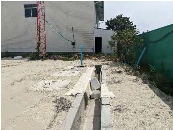
Trench-G (pipes diverted by WAMCO)
