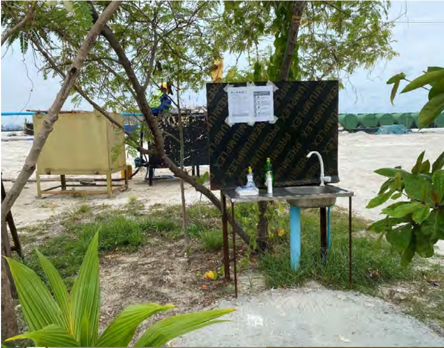
Hand wash stations and posters at the Harbour Rehabilitation site
