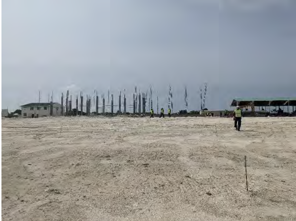
Project site compaction and grading
