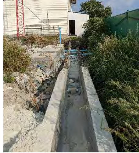
Trench-G (ask WAMCO to divert the pipes)
