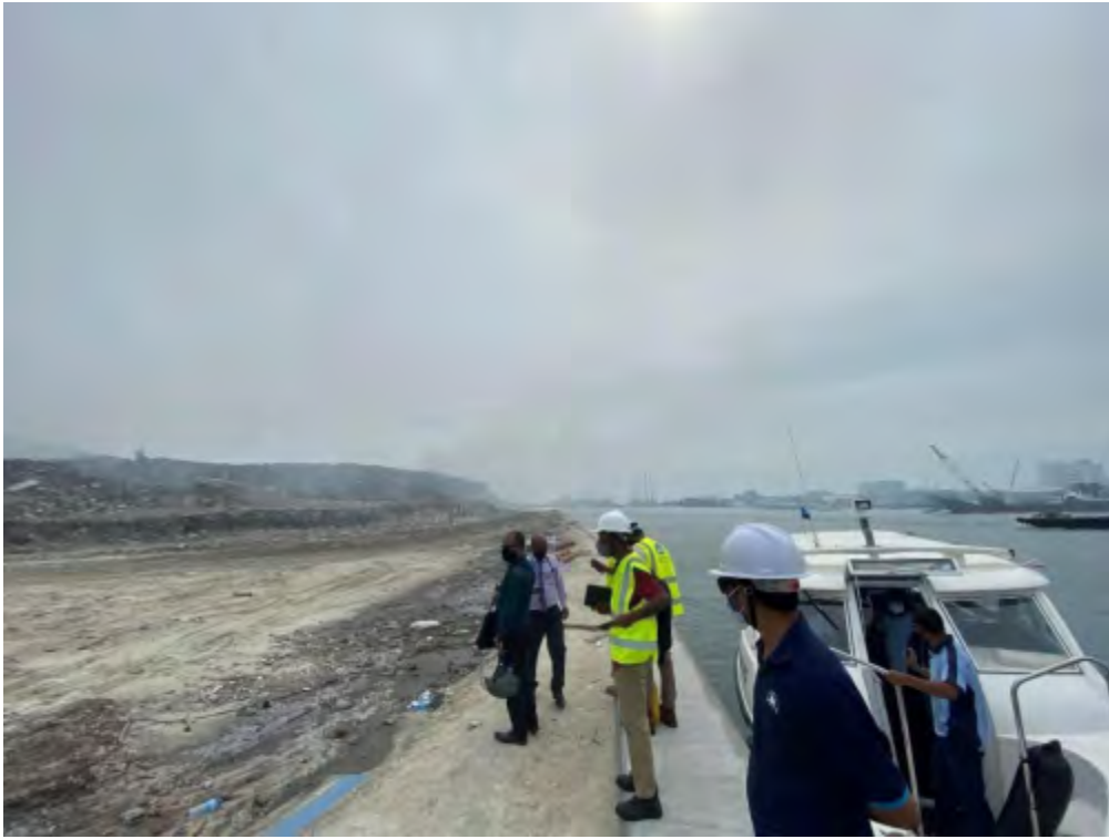
PMU and contractor teams at the Harbor Rehabilitation site
