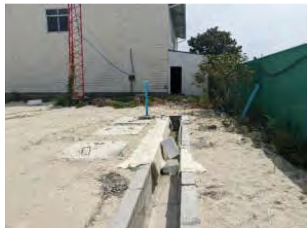
Trench-G (pipes diverted by WAMCO)
