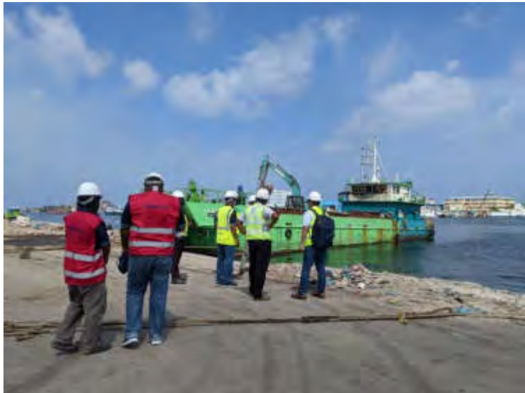
Inspecting ship ramp
