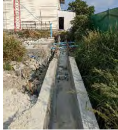
Trench-G (ask WAMCO to divert the pipes)
