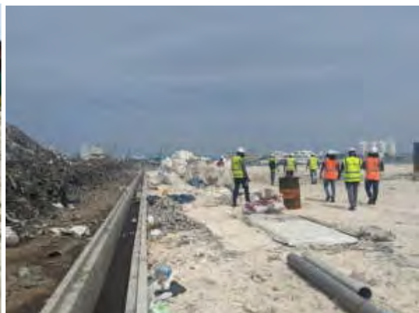
Trench-F (flooded with mud from the waste mound)
