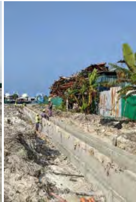
Trench-H (works on going)
