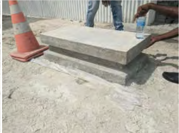
Concrete carriageway jointing sample
