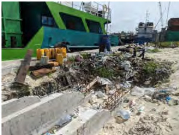
Trench-D (oil/sediment trap will be joined here)
