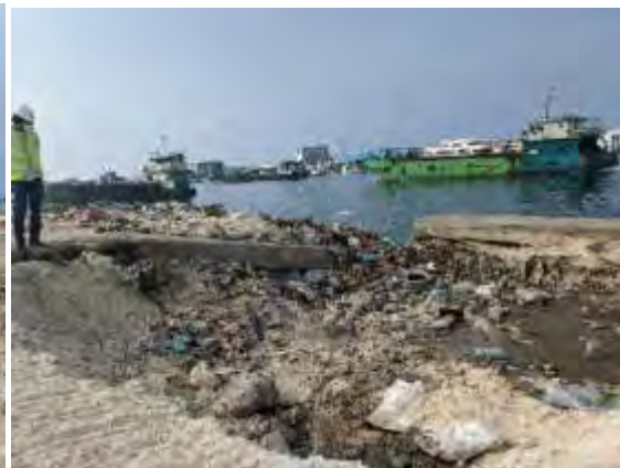
Ramp edge (careful of erosion under the ramp slab)
