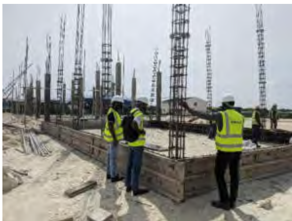
Admin Building foundation beam work
