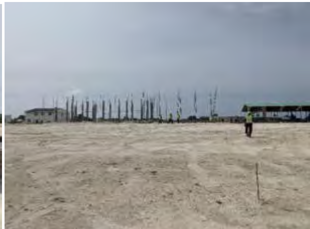
Project site compaction and grading
