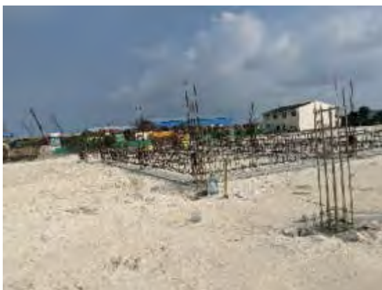
Admin Building foundation beam work
