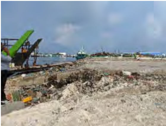
Ramp edge (the slope is pretty good)
