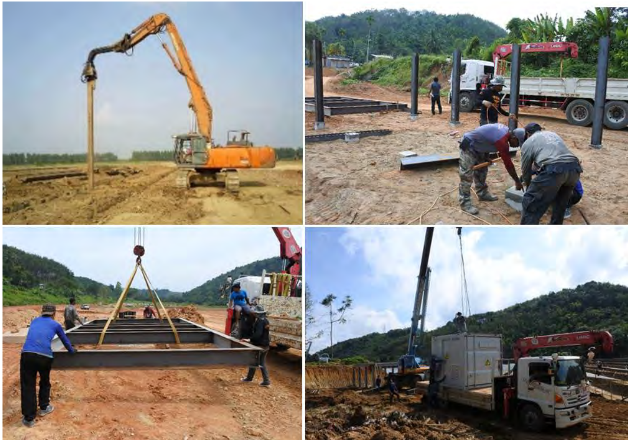
Figure 3.13: A typical scenario of piling by vibration and installation of transformers
