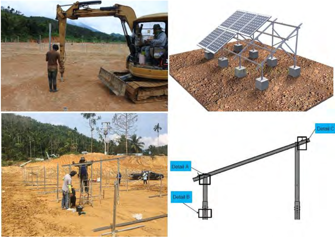
Figure 3.15: Installation of mounting structures
