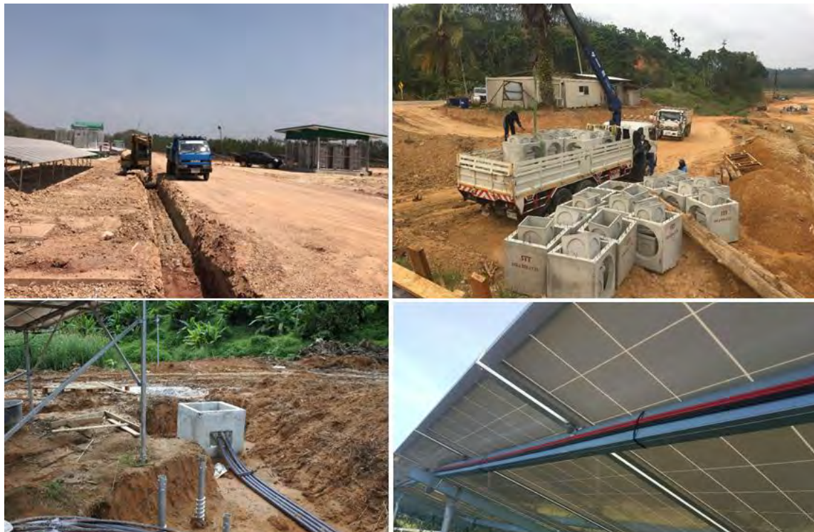
Figure 3.14: Cable connection and installation
