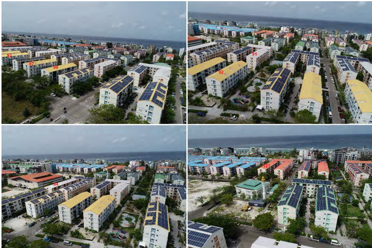
Figure 6.5: Rooftop installation area
