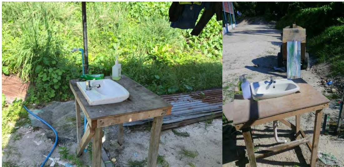
Figure 3 handwashing facilities at subproject sites
