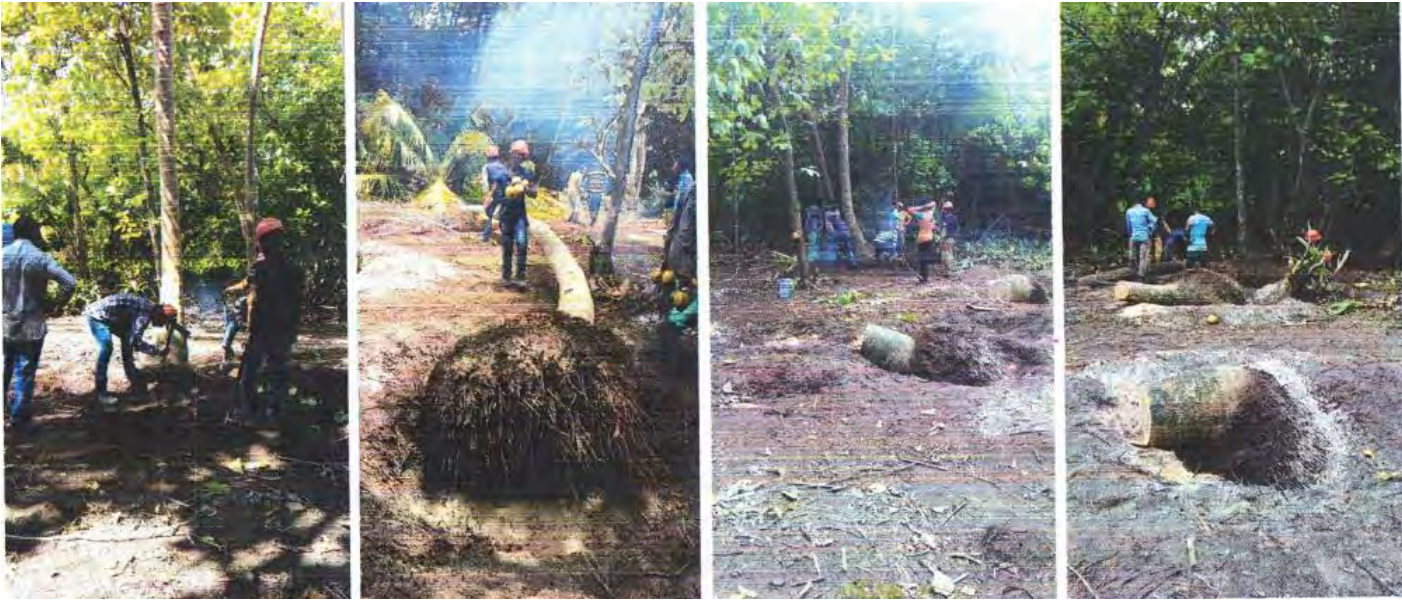
Figure 8 Vegetation removed from RO Plant Building Plot
