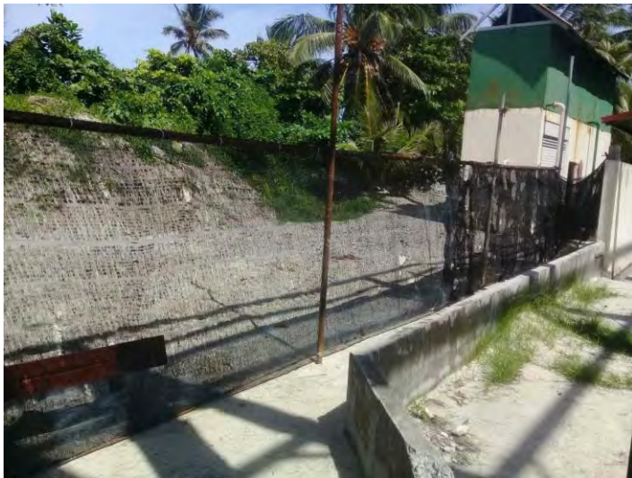
Figure 5 Site demarcation through fencing
