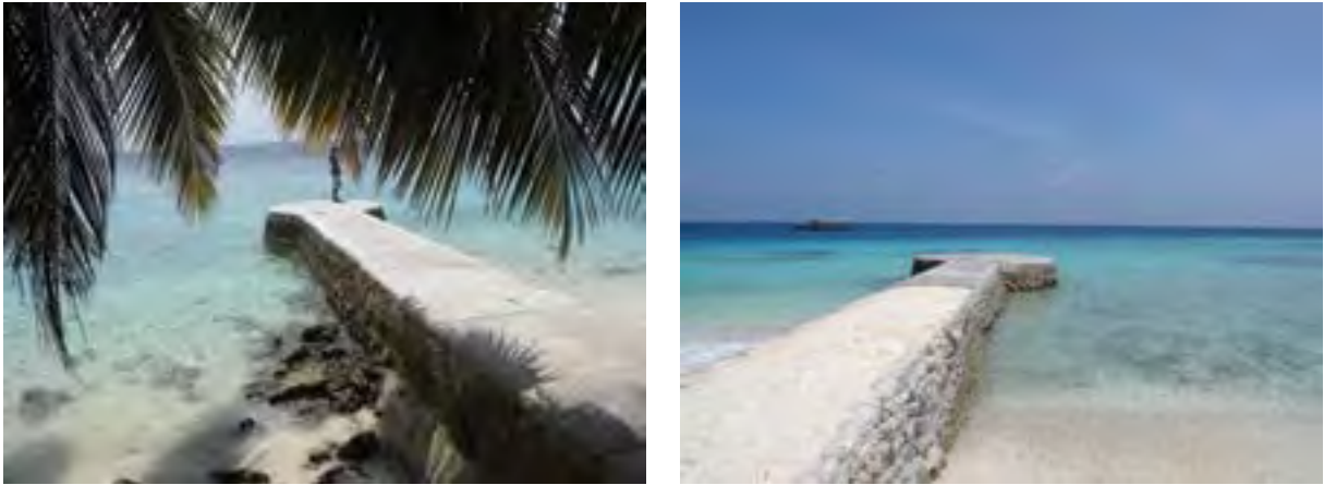
Figure 4.28 Sand cement bag and coral mound groynes in Sun Island Resort
