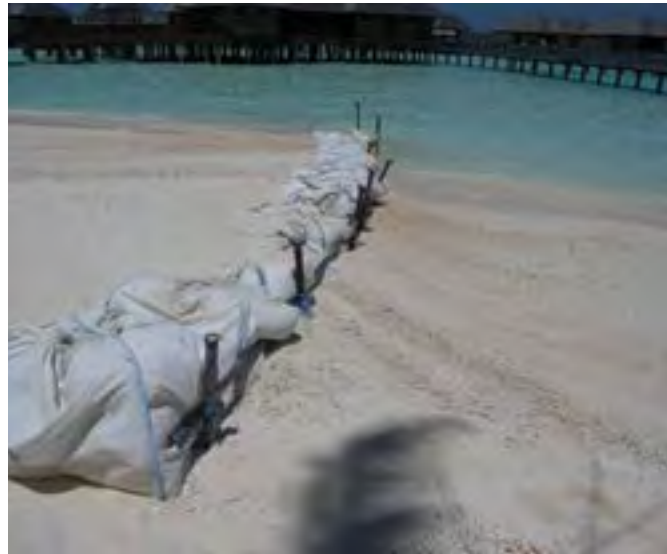
Figure 5.3 Temporary seawalls constructed in B. Royal Island and N. Irufushi Island
