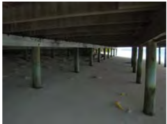
Figure 5.23 Use of stilts and retaining walls in Dh. Vilu Reef Resort
