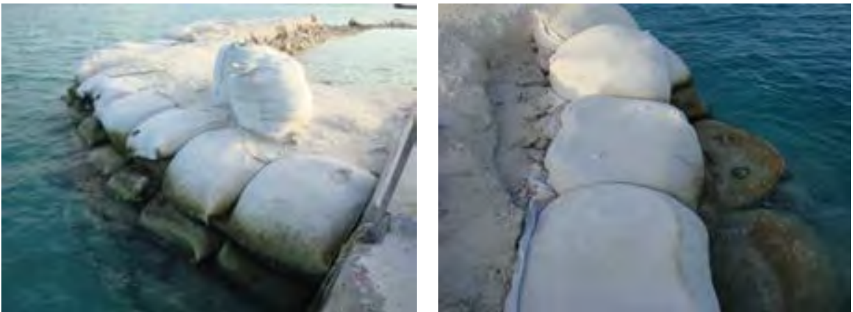
Figure 4.14 Adhoc seawalls in (clockwise from left) GA. Dhevadhoo , GDH Thinadhoo, GA Kolamaafushi and B. Eydhafushi
