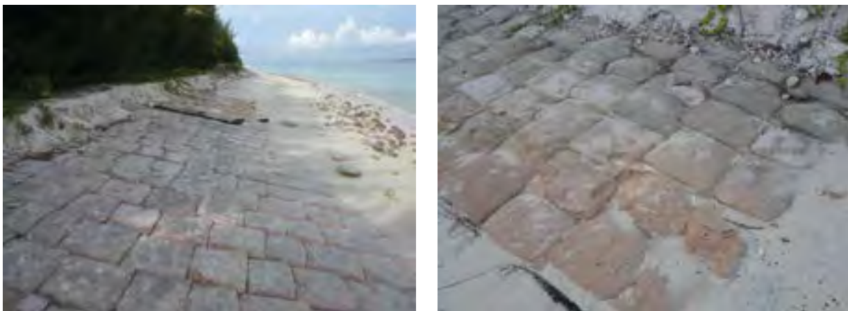
Figure 4.24 Generic revetment design – Sand-cement bags in Hulhumale’
