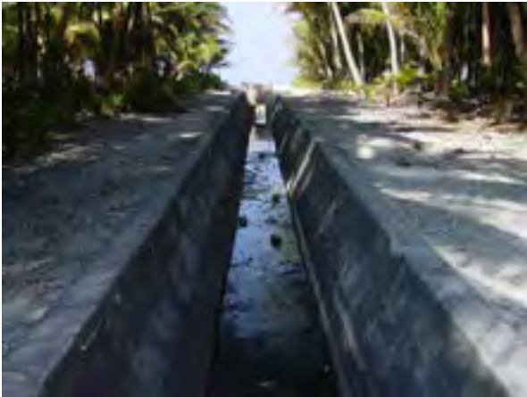
Figure 4.34 Rainfall flood mitigation measures in Ga. Viligilli
