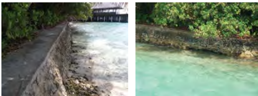
Figure 4.7 Examples of Seawall structures: semi-plastered coral mound seawall in Boduhithi
