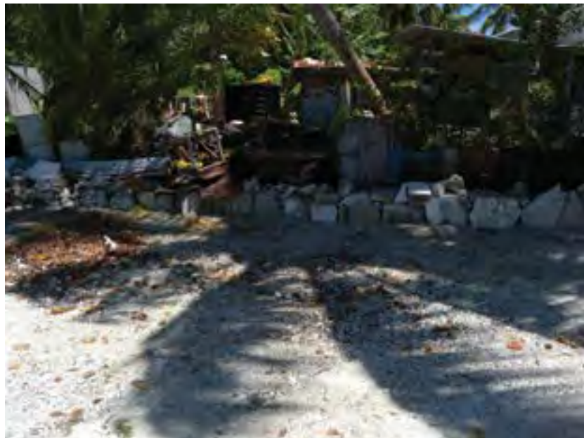
Figure 5.18 Use of both construction debris to protect properties from flooding in S. Feydhoo
