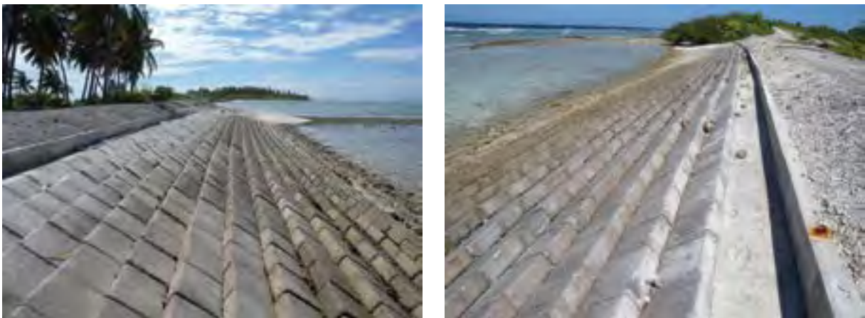
Figure 4.24 Generic revetment design – Sand-cement bags in Hulhumale’
