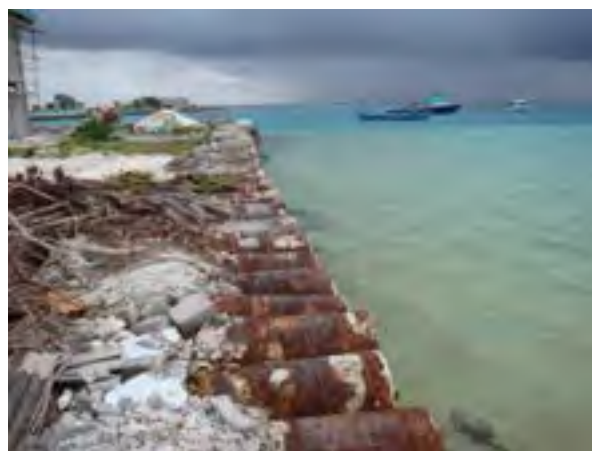
Figure 4.12 Examples of Seawall structures: 'Jumbo bags' in R. Dhuvafaru
