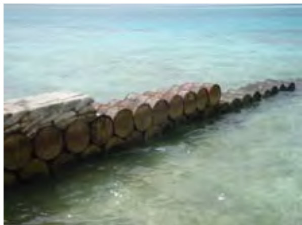
Figure 4.30 Groynes constructed concrete filled empty oil barrels in M. Maduvvari
