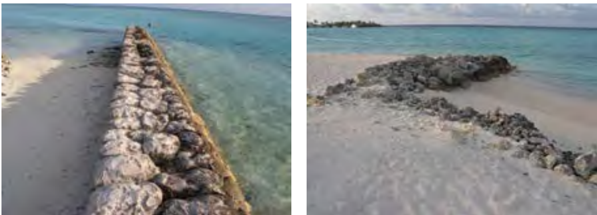
Figure 4.29 Groynes constructed from coral rubble in B. Reethi beach and AA Bodufolhudhoo
