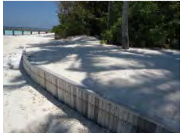
Figure 4.9 Examples of Seawall structures: unplastered sand cement bag seawall in M. Maduvvari and Sun Island Resort
