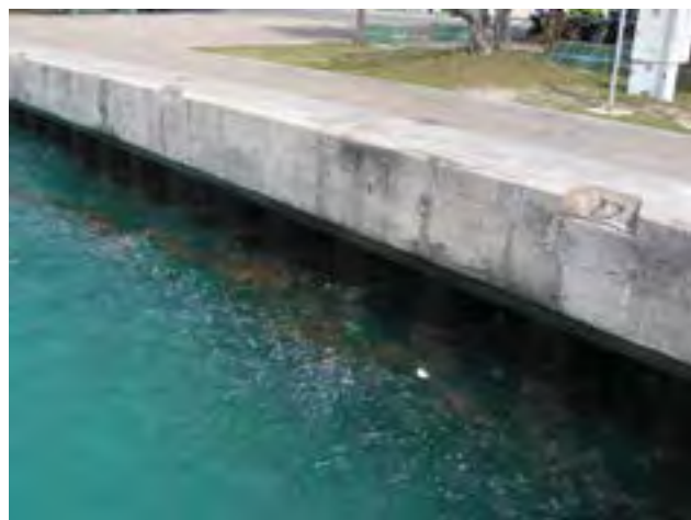
Figure 4.32 A modern quay wall in Hulhumale' constructed from sheet piles and concrete
