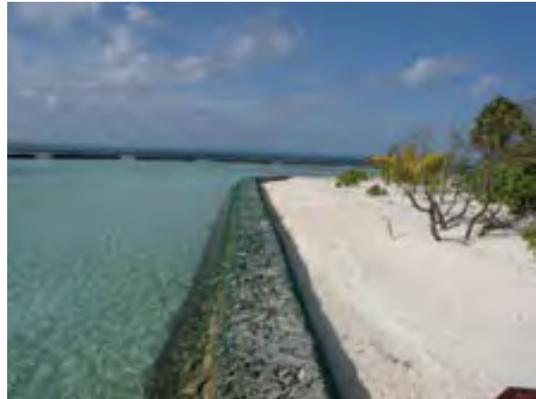
Figure 4.8 Examples of Seawall structures: unplastered coral mound seawalls in M. Maduvvari and Lh.
