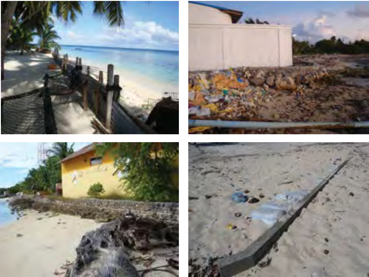
Figure 4.14 Adhoc seawalls in (clockwise from left) GA. Dhevadhoo , GDH Thinadhoo, GA Kolamaafushi and B. Eydhafushi
