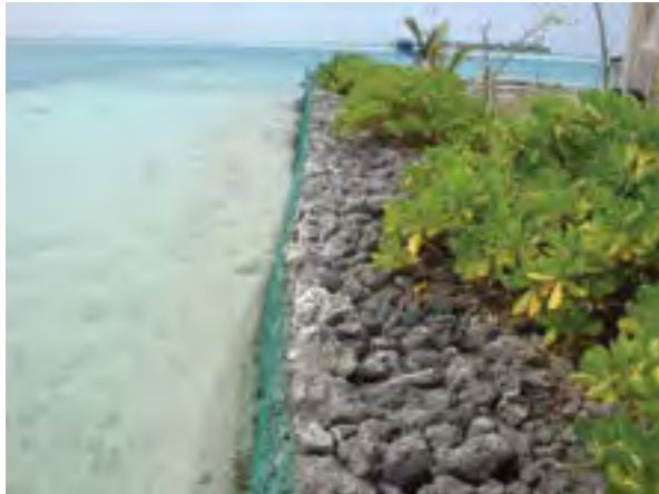
Figure 4.8 Examples of Seawall structures: unplastered coral mound seawalls in M. Maduvvari and Lh.
