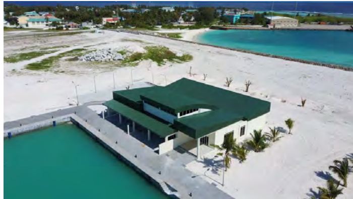
FIGURE 4 AERIAL IMAGE OF FERRY TERMINAL BUILDING
