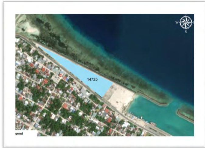
FIGURE 5 PV INSTALLATION AREA AT FEYDHOO HABOUR
