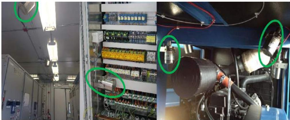
*Figure 4: Aerosol generator installation*
