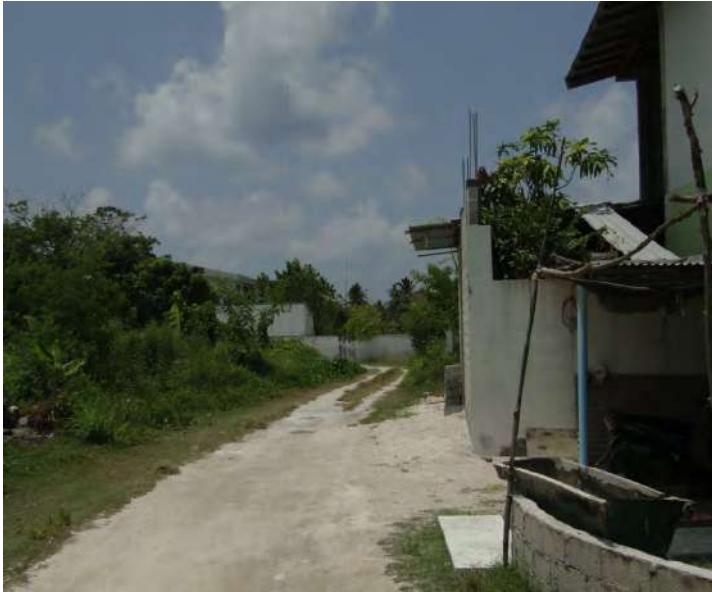
Flooding area – depth of flooding is around 0.30m
