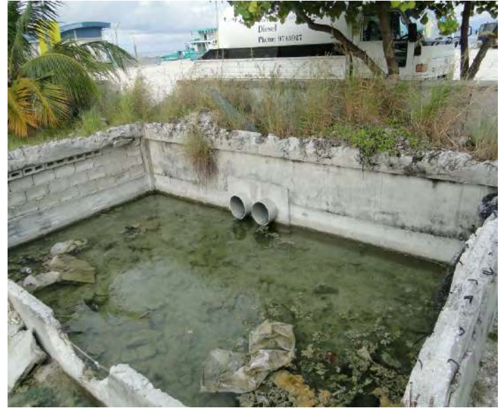
Existing drainage inlet – upstream of the sea
