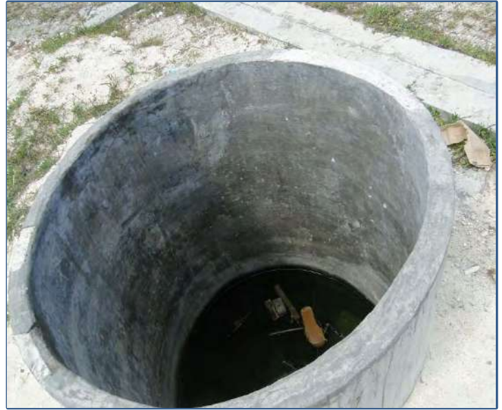
Observation from existing well to determine height of the ground tank
