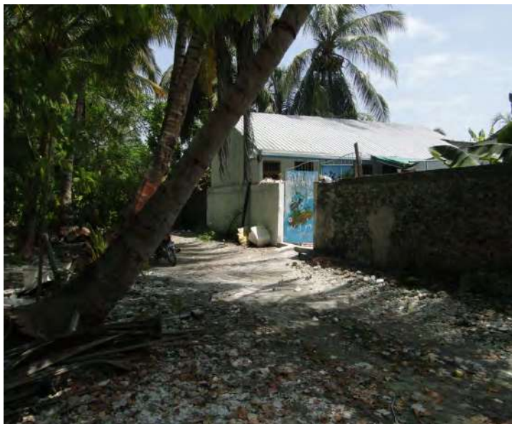
Houses are getting flooded about 0.30m
