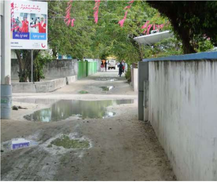
Water collected at junction. Closed by playground.
