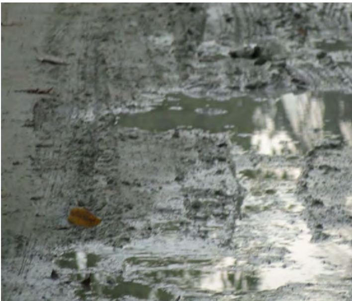
Low elevated areas along the link road to be filled to match natural slope
