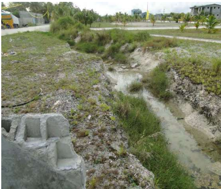
Earthen drain constructed by council
