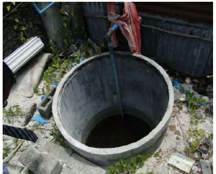
Well showing existing water table
