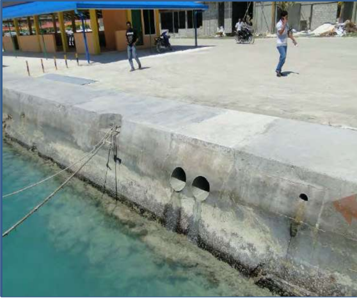
Flap gate to be constructed to prevent salt water intrusion in to inland area
