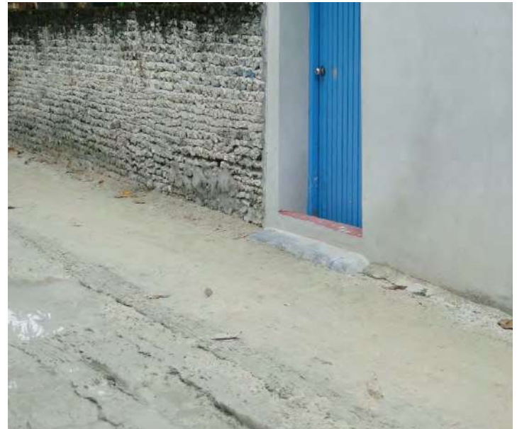
House entrance has been raised to protect from road floods
