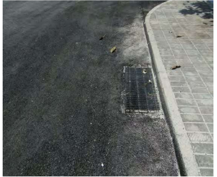
Newly constructed asphalt road with gully grating
