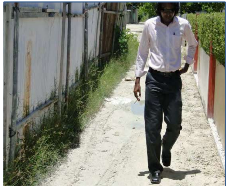
Flooding area without proper outfall
