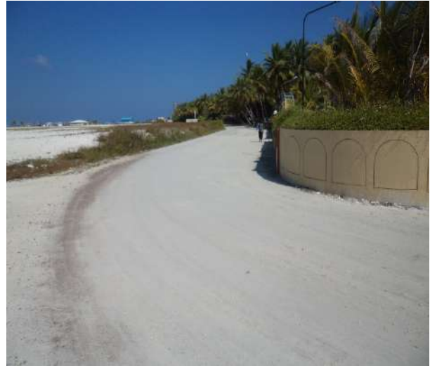
Existing road along the peripheral drain selected for the ground tank
