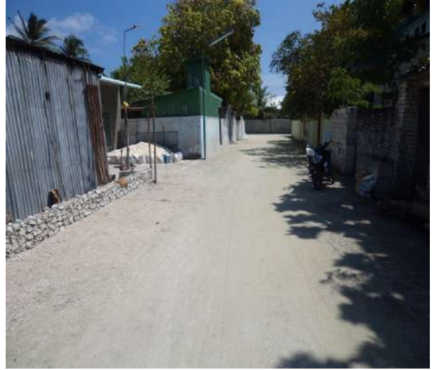
Lowest point flooding is taking place
