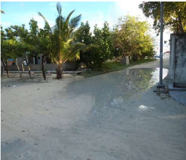
Inlet condition of the newly constructed shallow box culvert
