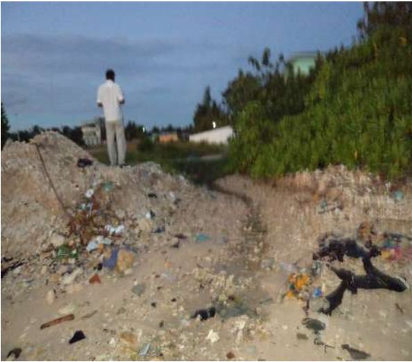
Downstream view of the existing earthen outfall Zone C
