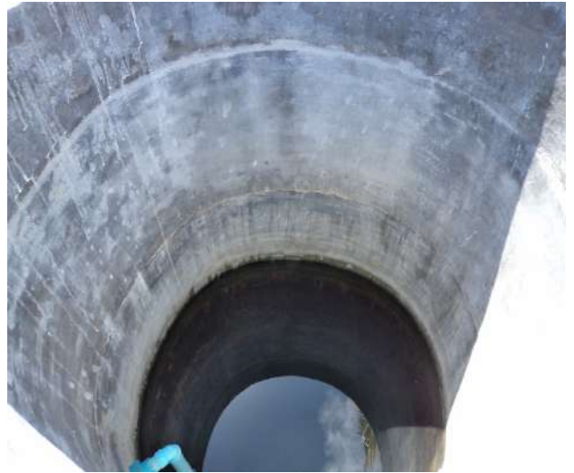
Water Level in the well during rainy period
