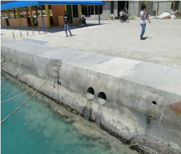
Existing emergency outlet location 01 Zone A
