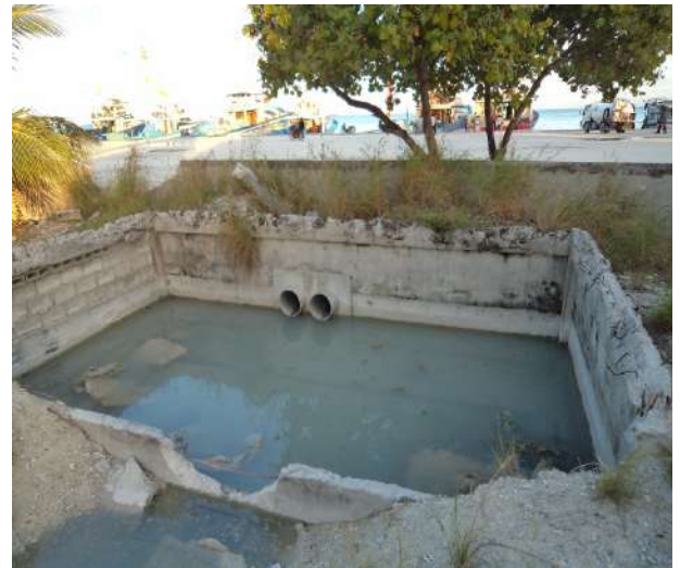
Inlet of the existing pipe culvert into sea – pilot project A
