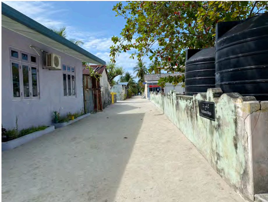
Figure 14: Access road condition
