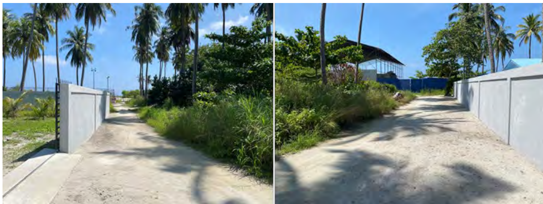
Figure 5: Access Road condition
