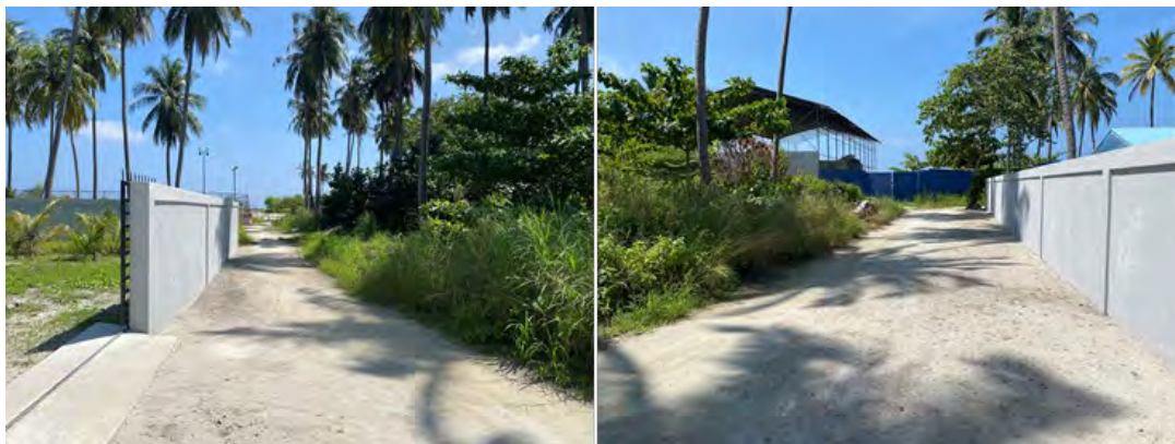
Figure 18: Access road condition
