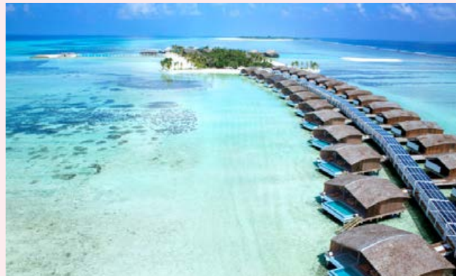
Figure 6-6: Solar PV array at Gasfinolhu (source: http://www.seattletimes.com )
