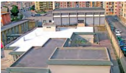
Cool Roof through white Coating
