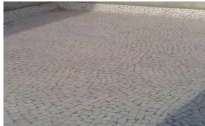
Cool Roof through China Mosaic
