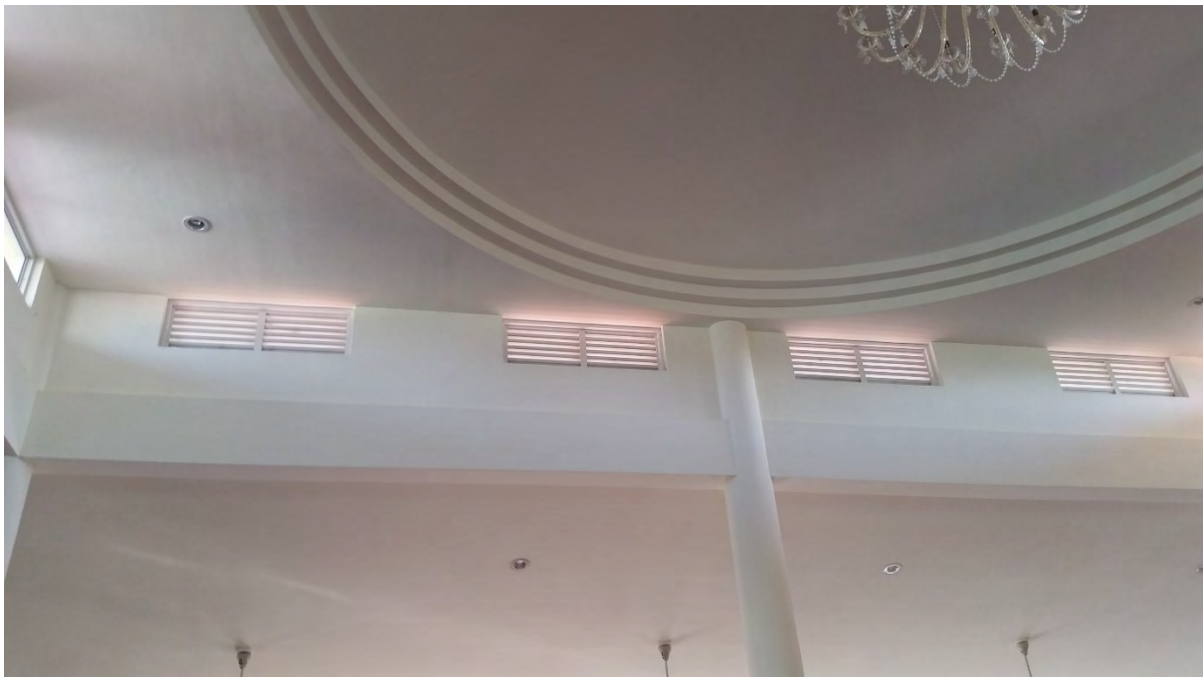
Figure 2-3: Relatively small area for air to escape at high level
