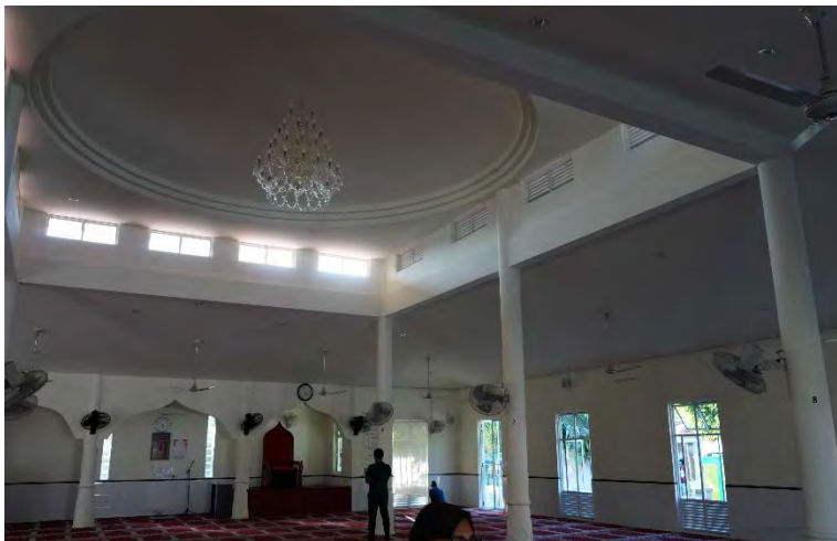
Figure 1-15: High level openings within the Masjid-ul Sidheeq
