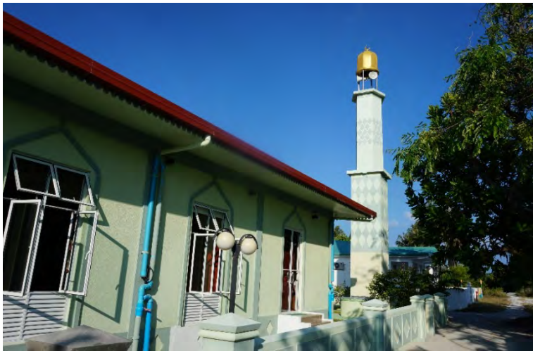
Figure 1-14: Existing windows at Masjid-ul Sidheeq
