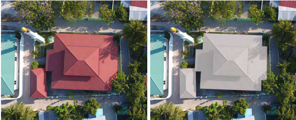
Figure 2-9: Existing (figure left) and recommended (figure right) roof colour
