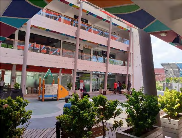
Figure 172– Image showing C shaped building block
