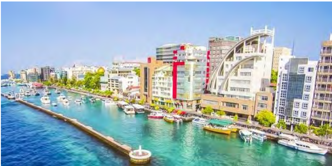
Images showing sea facing commercial buildings
