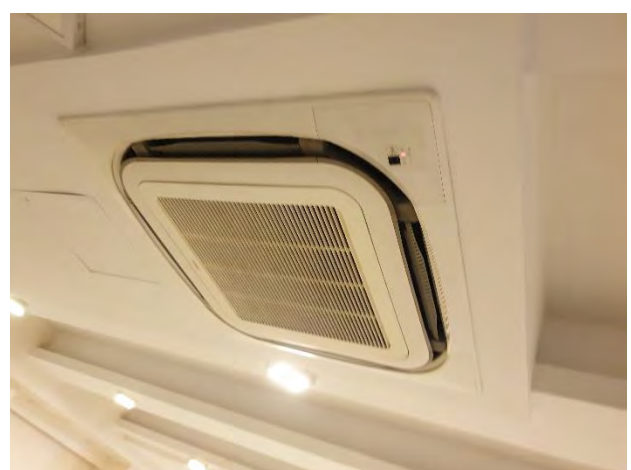
Figure 208– Images showing indoor ceiling mounted units of VRV system in the banquet areas
