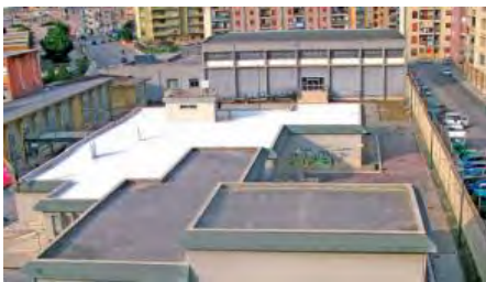
Cool Roof through white Coating
