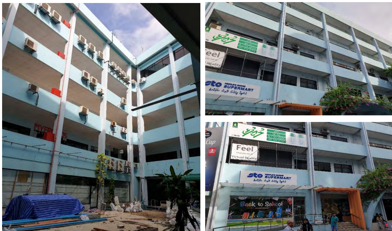
Figure 162 –View of the building
