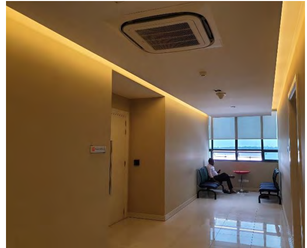
Figure 116– Image showing usage of Artificial lighting in the common area .
