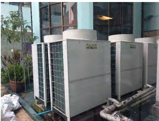
Figure 170– Images showing indoor ceiling mounted units and outdoor units of VRV system in supermarket
