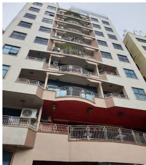
Figure 189 –View of the Residential Building
