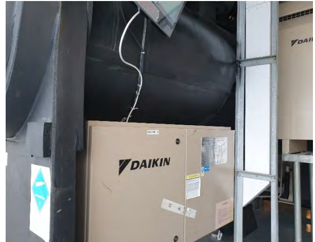
Figure 121– Image showing Daikin 400 TR water-cooled Chiller
