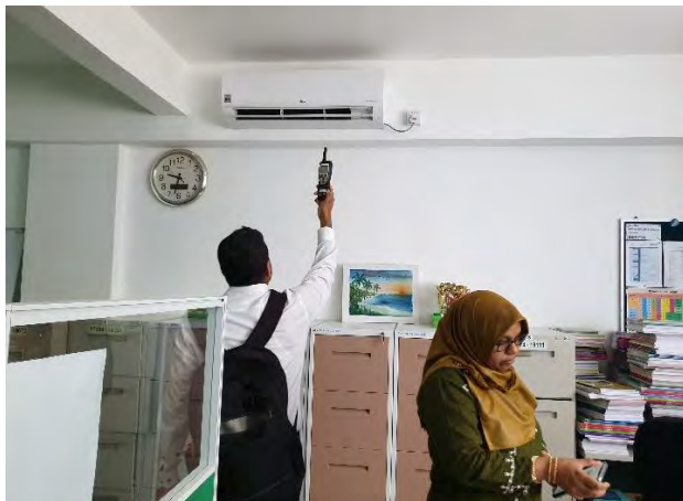
Figure 106– Image showing high wall unitary air conditioners in staff rooms
