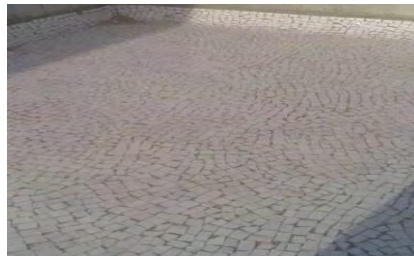
Cool Roof through China Mosaic
