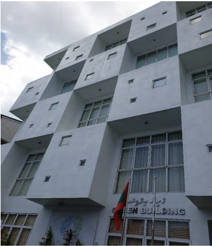
Figure 86 – Front View (East) of the building
