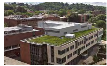
Cool Roof using Landscaping
