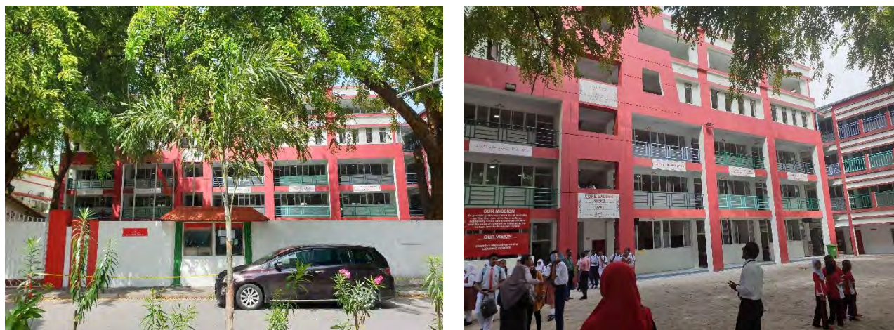
Figure 136 – Front View of the building
