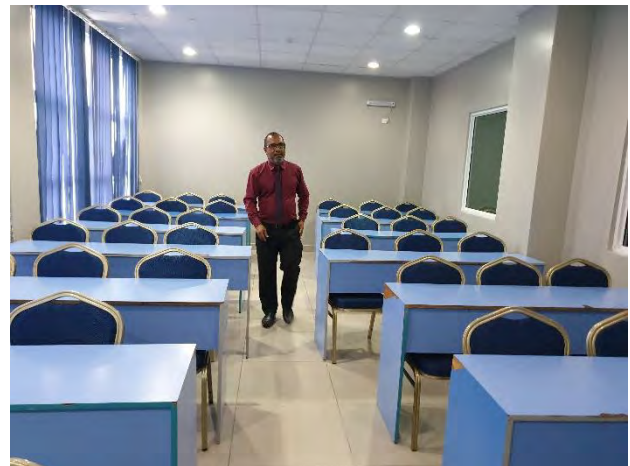
Figure 158– Image showing LED lighting in classrooms
