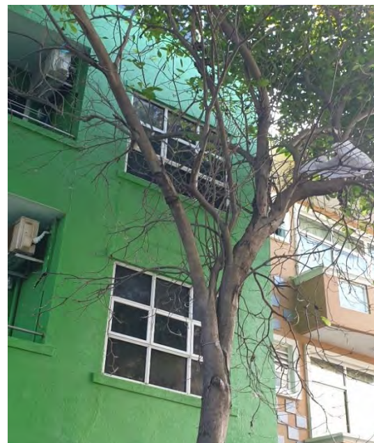
Figure 217 –View of the building
