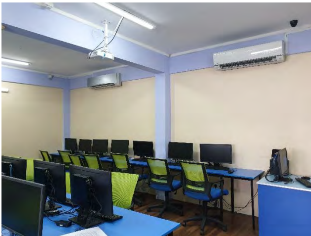
Figure 159– Image showing wall mounted AC in the computer lab in old building
