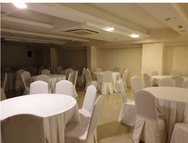
Figure 208– Images showing indoor ceiling mounted units of VRV system in the banquet areas
