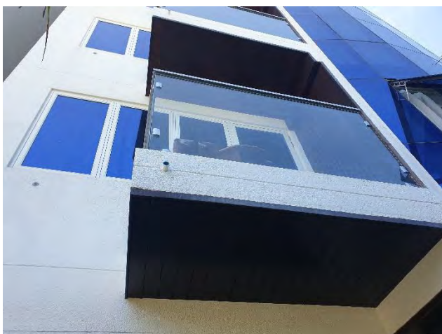
Figure 211– Images showing shading provided by the balcony
