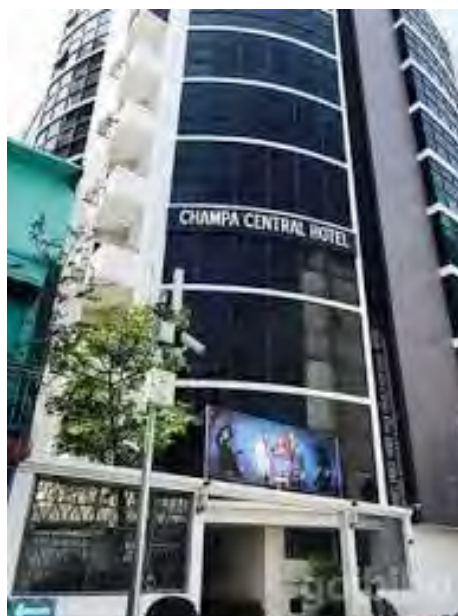
Figure 205 –View of the building
