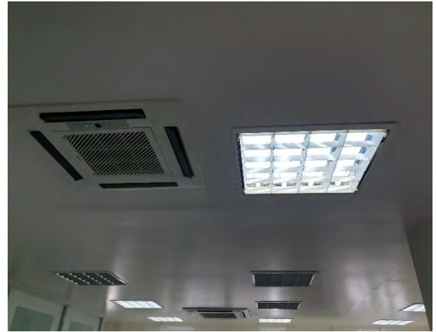
Figure 188– Images showing wall and ceiling mounted AC in the office
