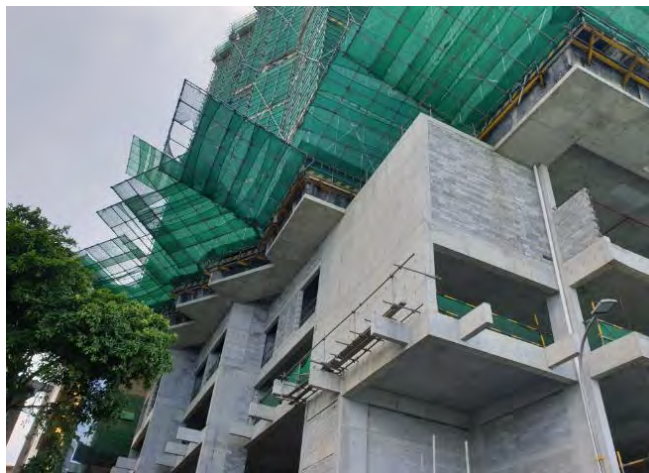
Figure 17: Image showing Masonry blocks used in construction
