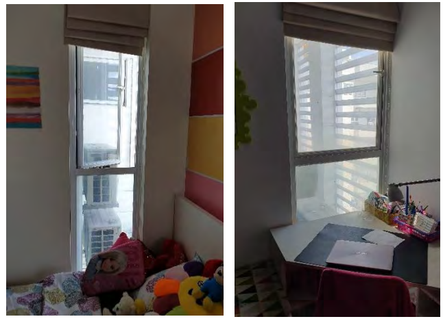
Figure 193 –Images showing recessed windows in the bedroom
