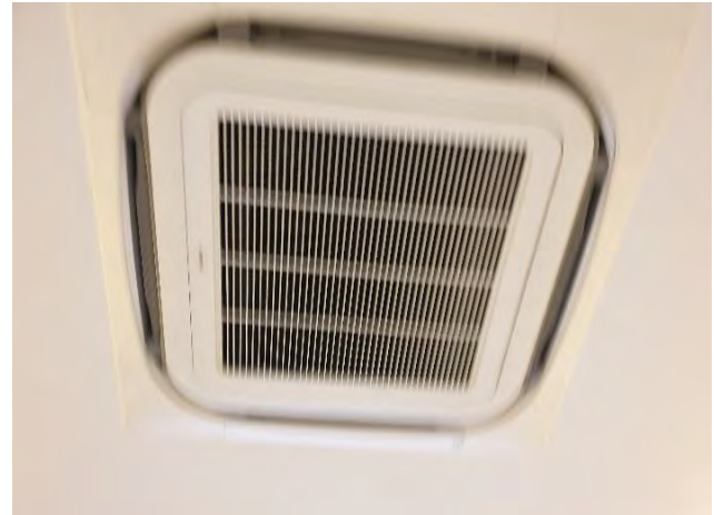
Figure 151– Image showing indoor ceiling mounted units of VRV system in workspace
