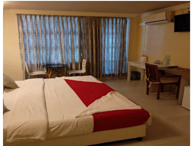
Figure 224– Image showing wall mounted split ACs in guest rooms
