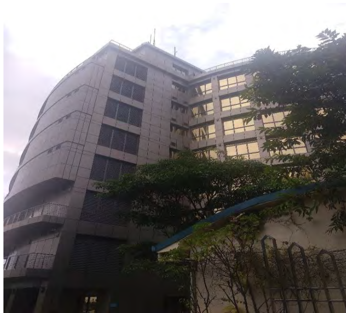
Figure 108 – STO Head Office building
