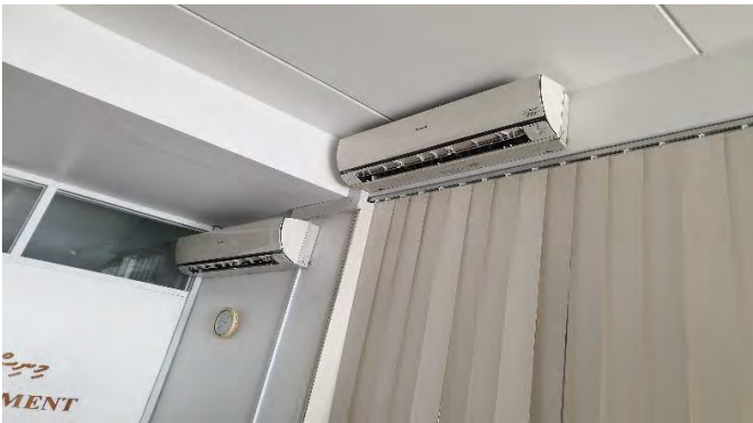
Figure 95– Image showing high wall unitary air conditioners
