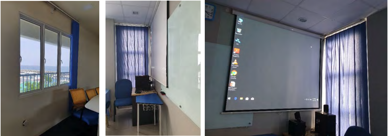
Figure 156 – Images showing use of high Window to wall ratio and blinds to avoid glare
