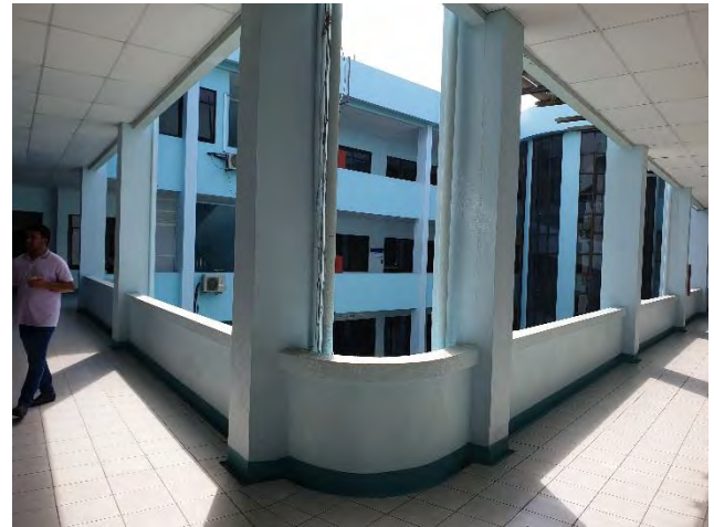
Figure 166 – Images showing shading by projecting balconies
