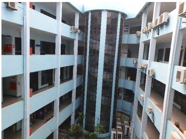
Figure 163– Image showing trapezoidal structure of the building
