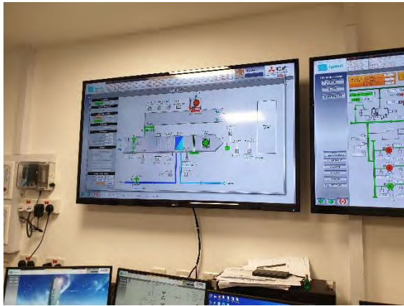
Figure 123– Images showing Building Management System (BMS)
