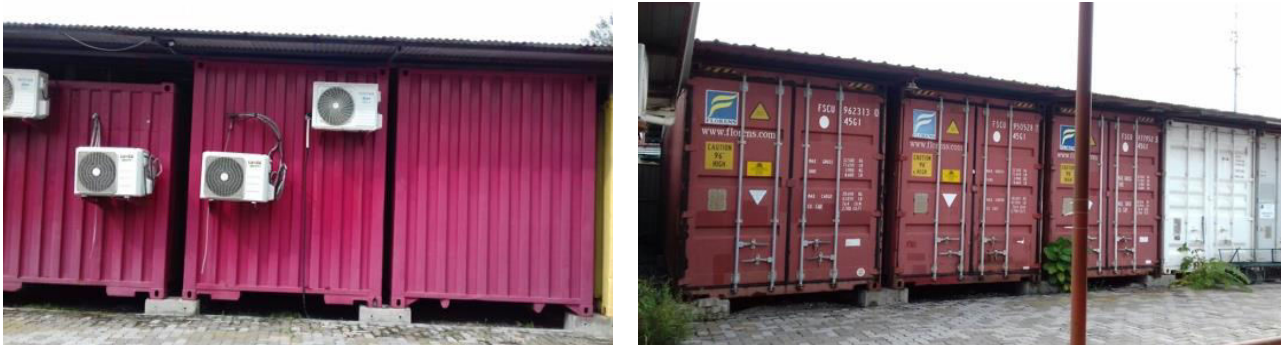
Figure 18: Reefer containers in the bonded warehouse of Maldives customs used to store products imported
