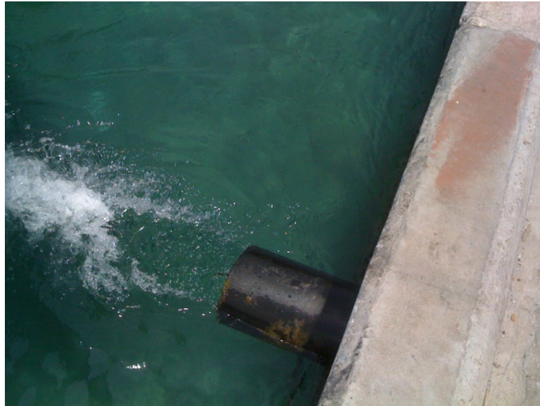
Figure 3.5: A brine outlet discharging to sea in Male' southern side harbour basin (Land and Marine Environmental Resources Group, 2010)
