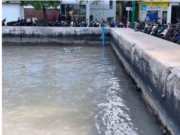
Figure 4.4: Northeastern harbour basin of Male' where groundwater from construction sites is discharged is often seen contaminated with dirty water. (Source: Authors)
