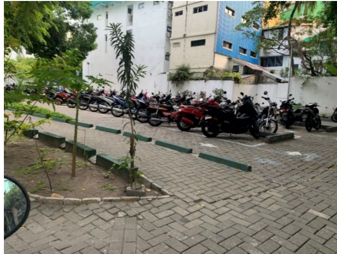
Figure 2.4: A motorbike parking zone in Male' where paved using interlocking paver blocks – (Source: Authors)
