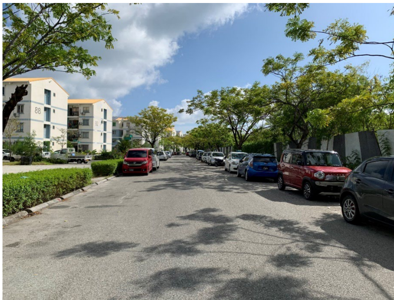
Figure 2.12: Bioretention systems or bioswales located on either side of the roadways in Hulhumale' allows drainage and filtration of rainwater before it infiltrates into the ground. (Source: Authors)
