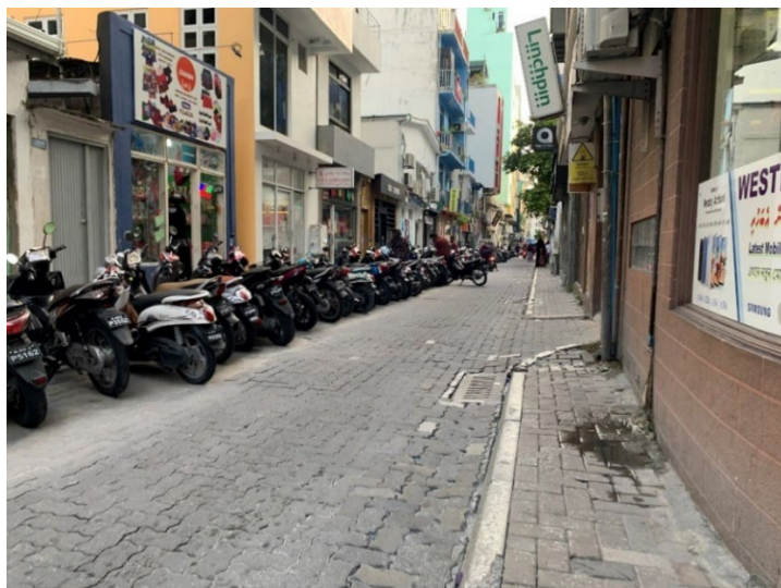
Figure 2.2. A paved road in Male' where vehicles are parked on the left side and catch pits are installed for drainage. This setup is different for a less-developed island in the Maldives – (Source: Authors)
