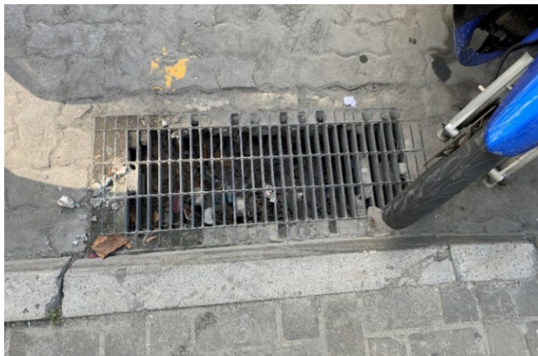
Figure 2.5: A stormwater catch pit located on the roadside of Male' city, seen filled debris and trash – (Source: Authors)
