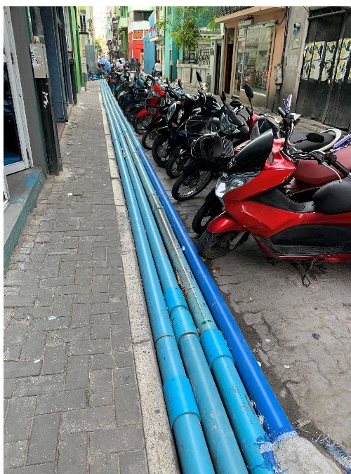
Figure 4.2: Discharge end of dewatering discharge pipes laid over the southwestern quay wall of Male'. (Source: Authors)
