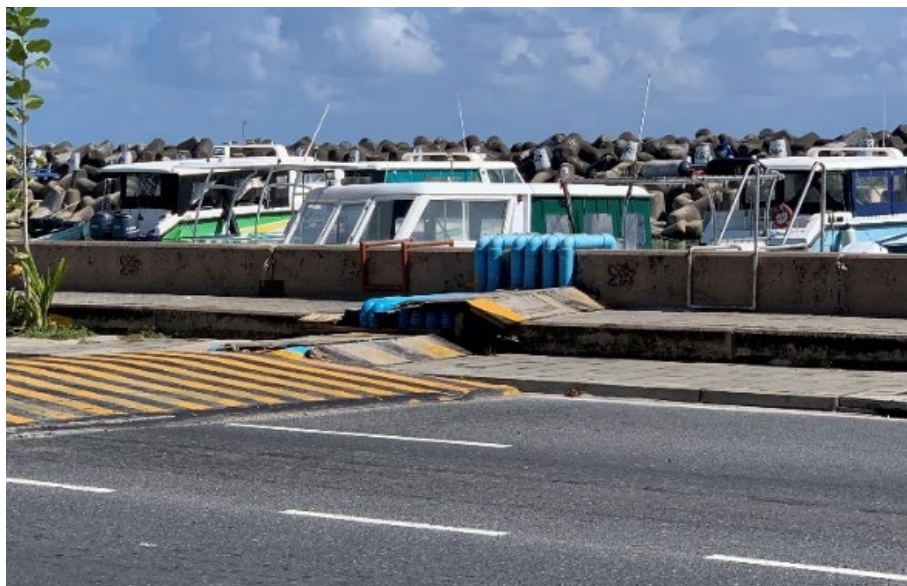
Figure 4.2: Discharge end of dewatering discharge pipes laid over the southwestern quay wall of Male'. (Source: Authors)
