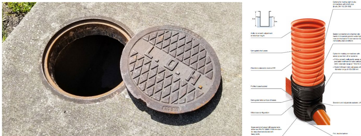
Figure 1.19. Photograph of a typical sewer manhole with the cover removed for inspection (left) and the details of the corrugated shaft pipe (right) – (Source: https://bcfocus.com/global-sanitary-manhole-covers-market-2020-industry-future-growth-key-player-analysis-and-forecast-2025/ , & http://www.ekoma.net.pl/oferta/735/tegra-425.html )
