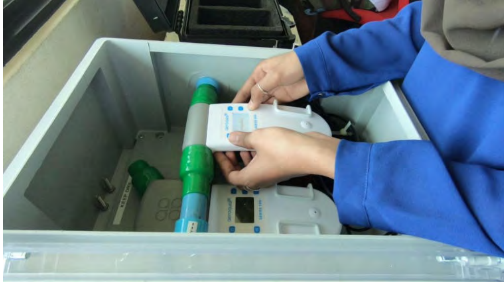
Figure 1: Air Quality monitoring station with two Aeroqual Series 500 monitors
