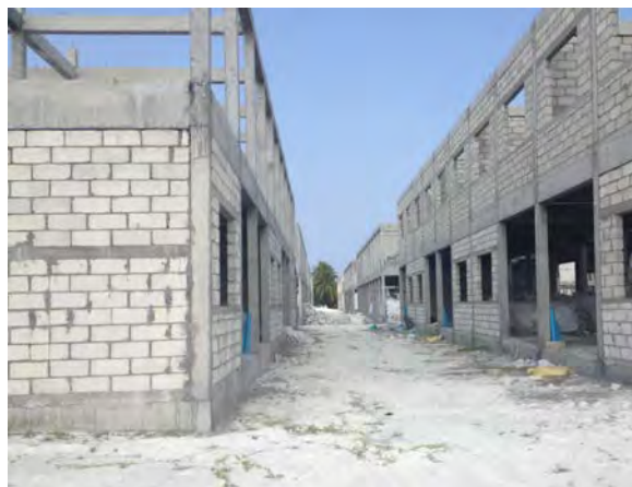
FIGURE 6 ROW HOUSES UNDER CONSTRUCTION AT THE NEWLY RECLAIMED LAND (VELIGANDU)
