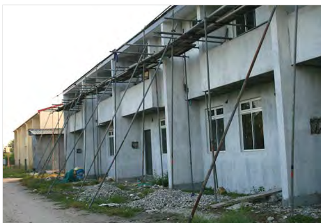
FIGURE 5 ROW HOUSES UNDER CONSTRUCTION AT THE NORTH SIDE WETLAND LAND AREA
