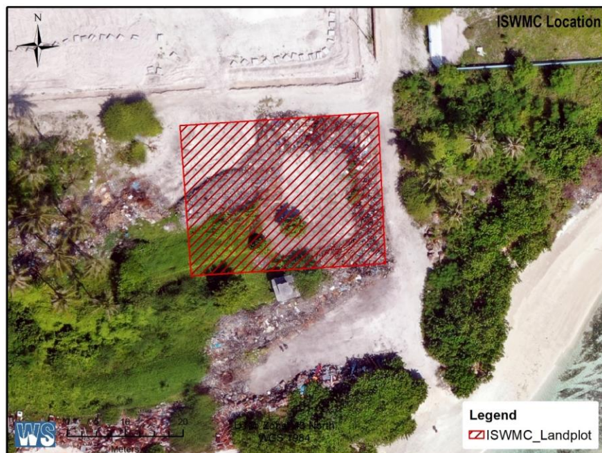
Figure 4: Closeup of site boundary overlaid over a drone photo taken on 21 January 2021.
