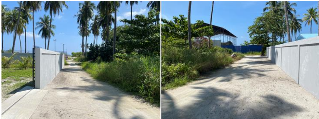
Figure 17: Access road condition
