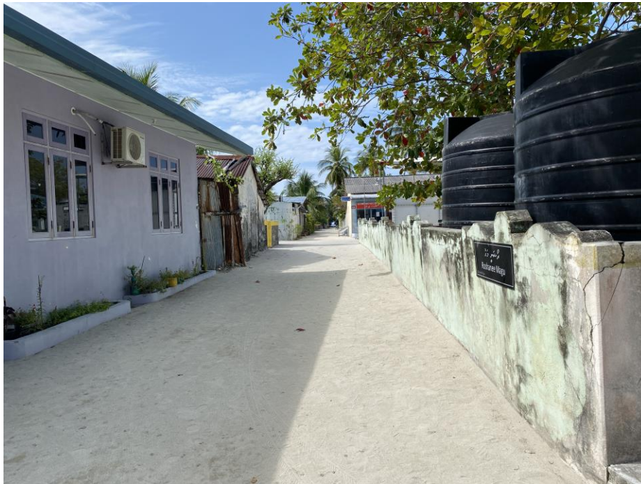
Figure 13: Access road condition
