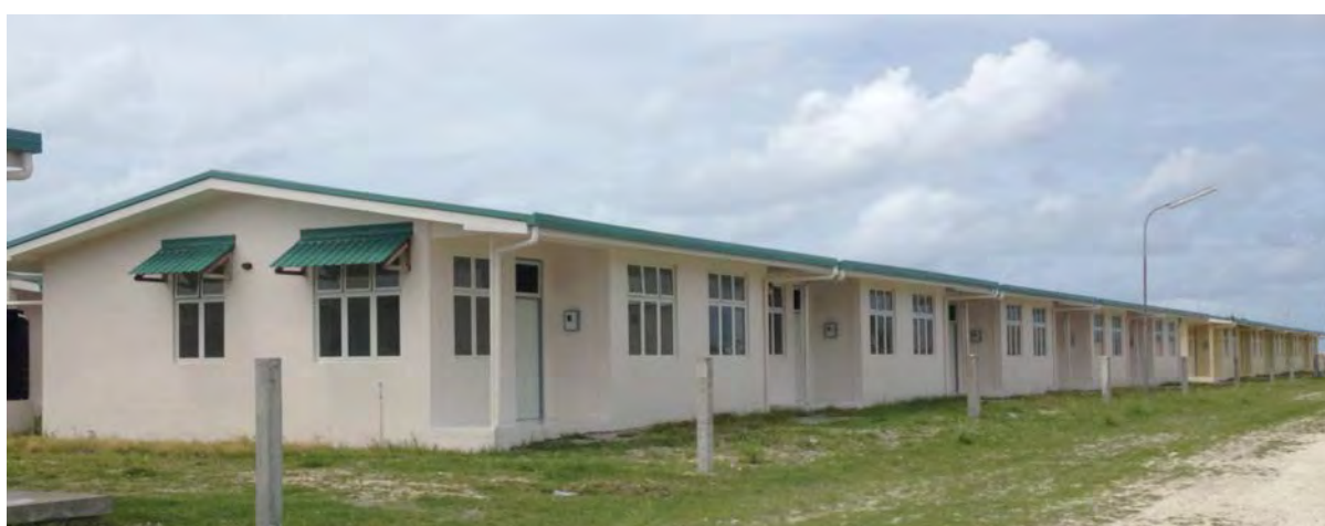
FIGURE 2 SINGLE STORY HOUSES, PROVINCE HOUSING DEVELOPMENT PROJECT
