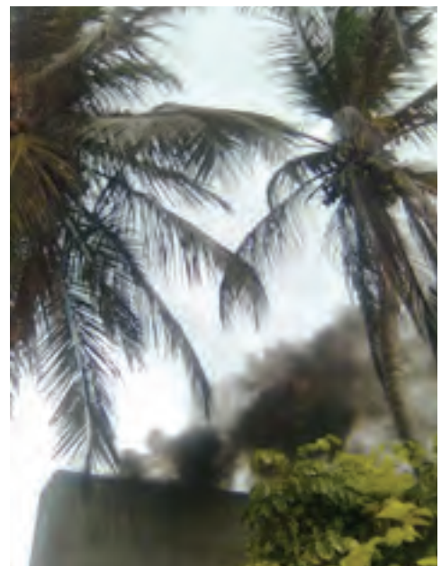
Black smoke emitted from a small powerhouse
