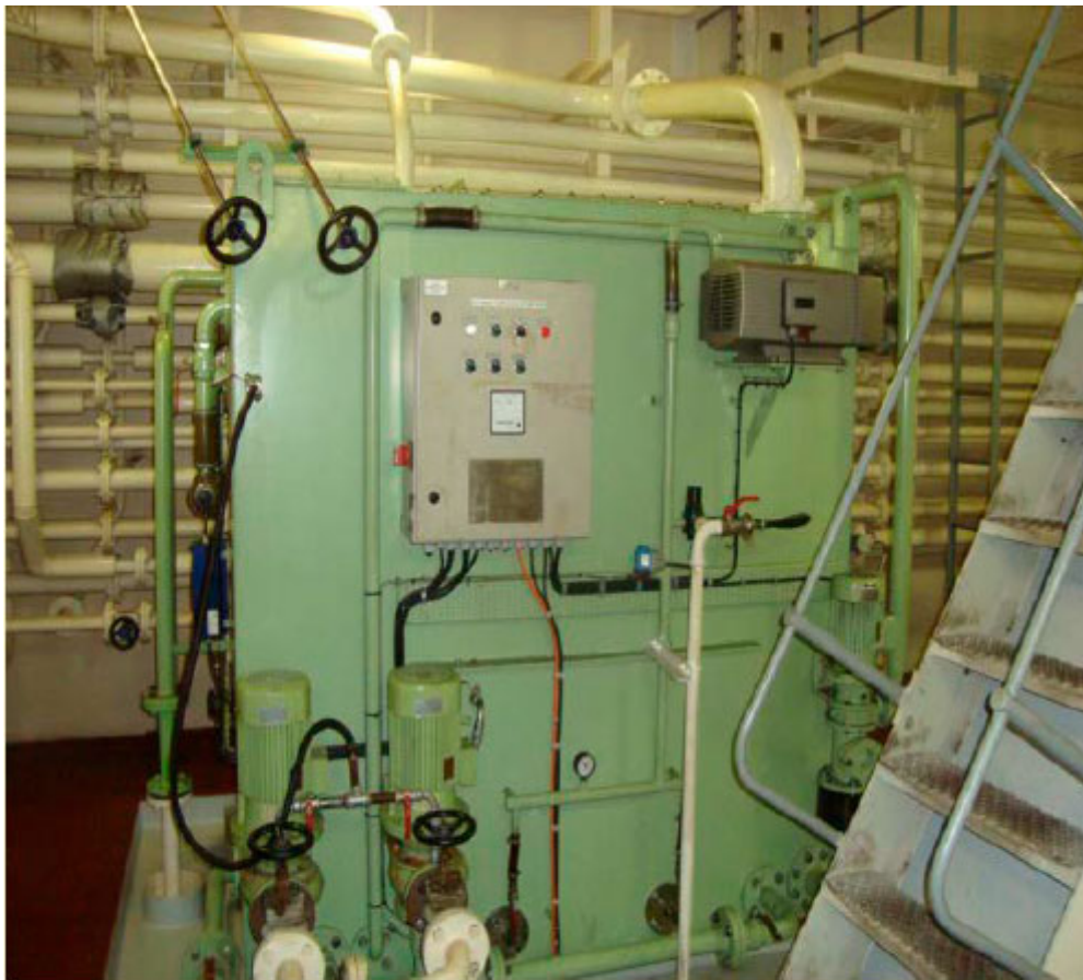
Sewage Treatment Plant
