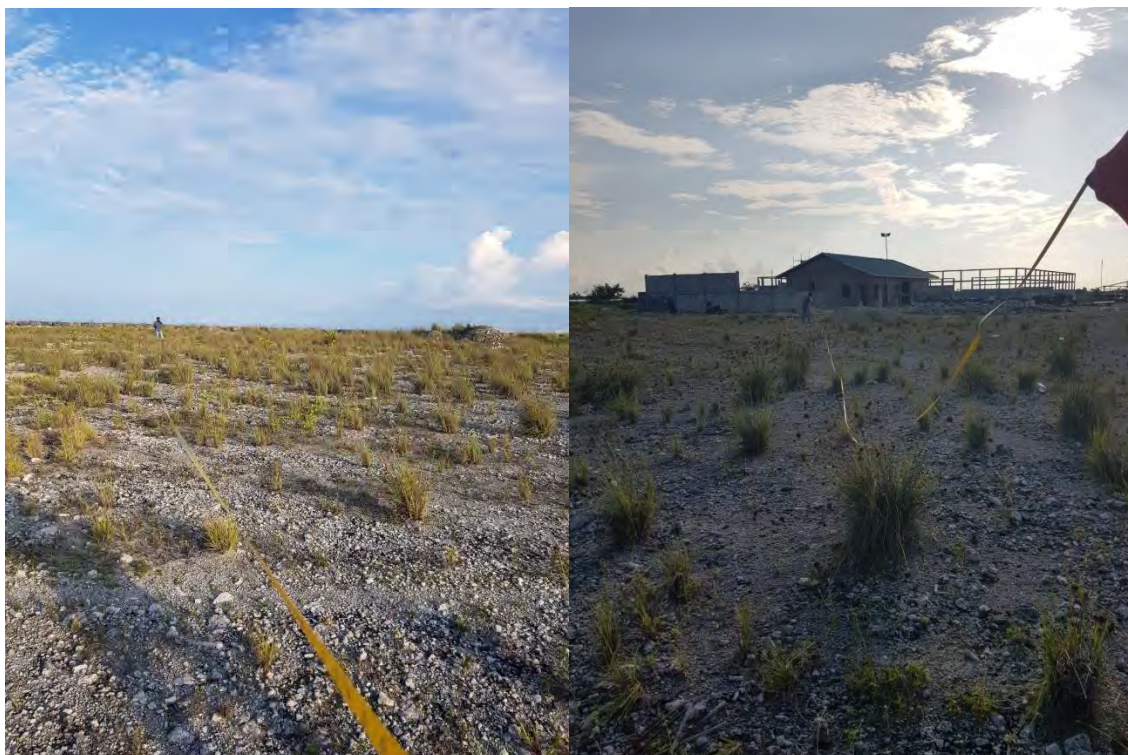
Figure 6 Site surveying works
