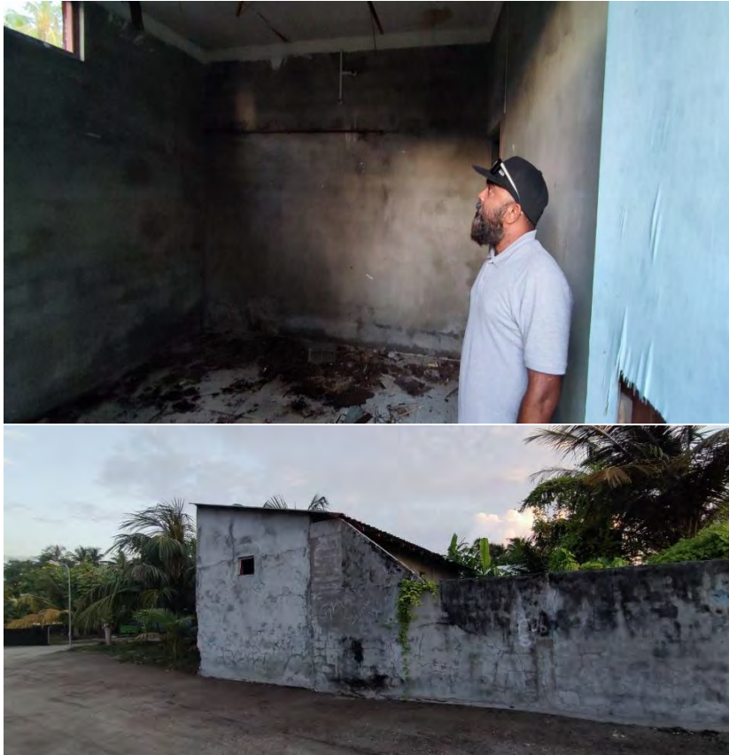
Figure 4 Material Storage Room
