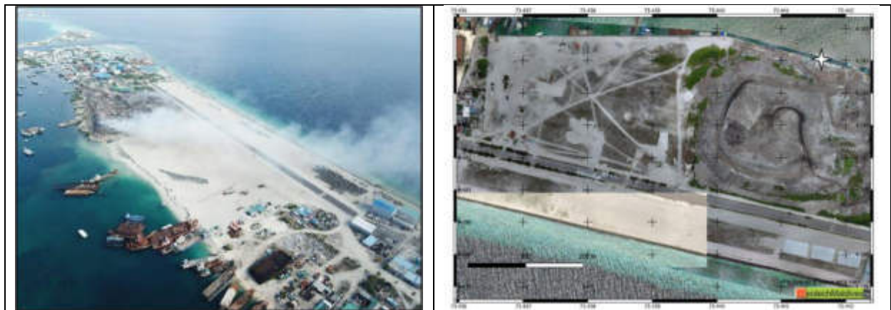
Figure 12: WtE Site in 2019 (left) and in 2022 (right)
