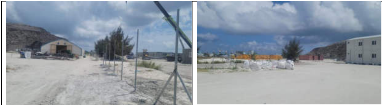
Figure 14: fence and office temporary buildings
