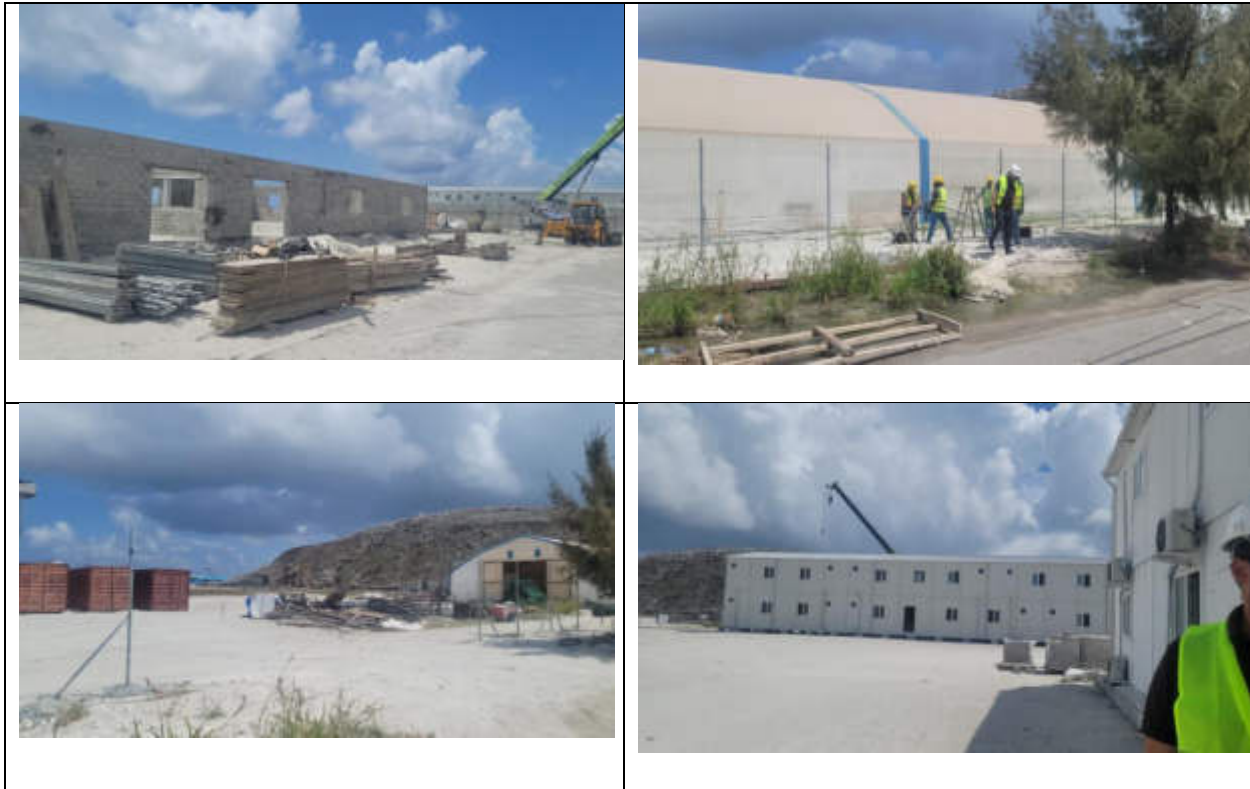
Figure 13: Progress of construction camp accommodation site office and admin buildings
