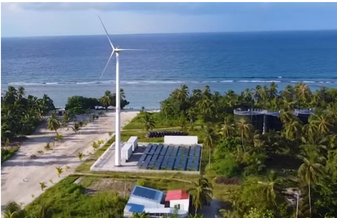
Wind - Solar photovoltaic and Battery Energy Storage system installed at K. Kaashidhoo Island.
