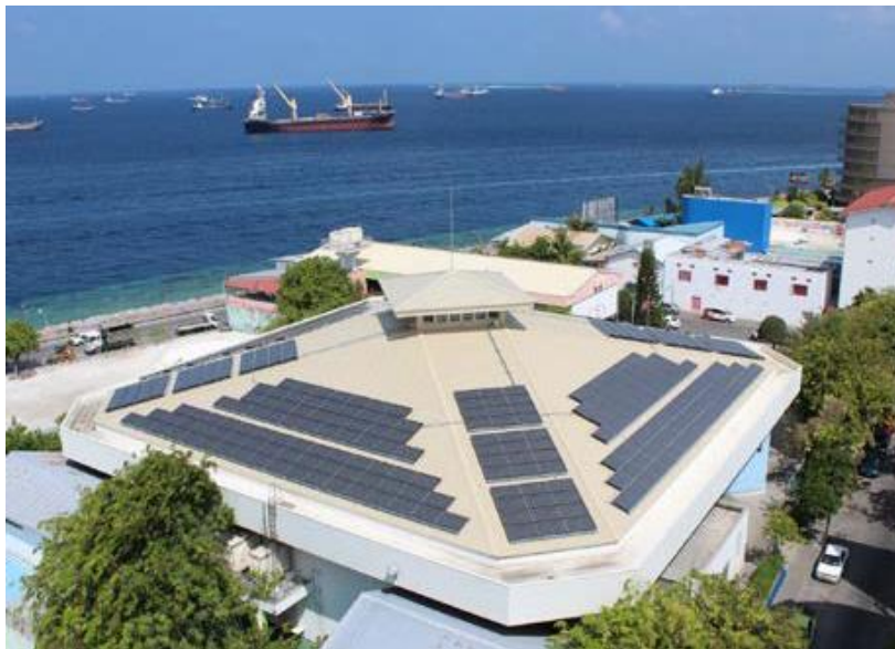
A 100 kilowatt peak solar PV system installed at Maldives Center for Social Education in Male' (photo by Ministry of Environment)
