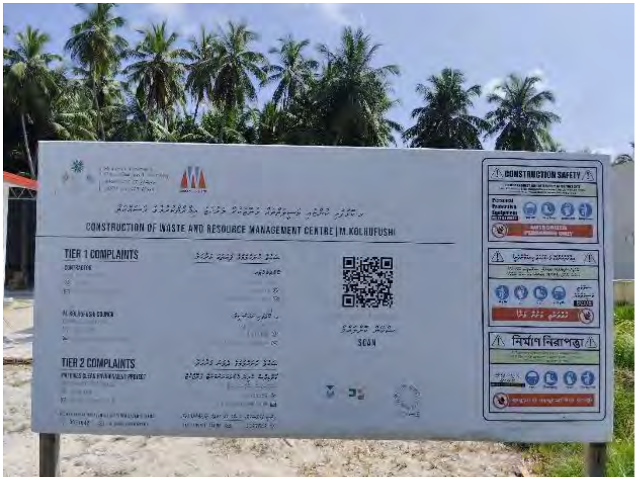
Figure 7. GRM board displayed at project site
