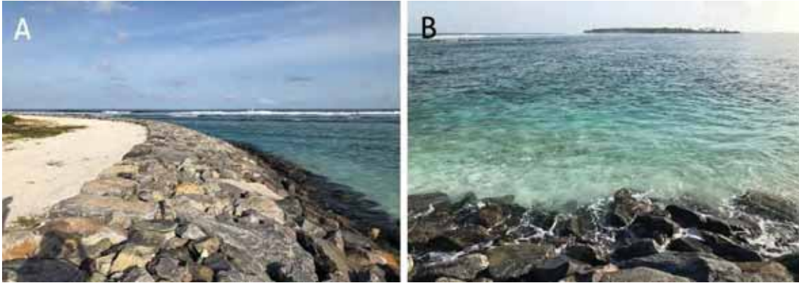
Figure 12: (A) and (B) Revetment close to the project area
