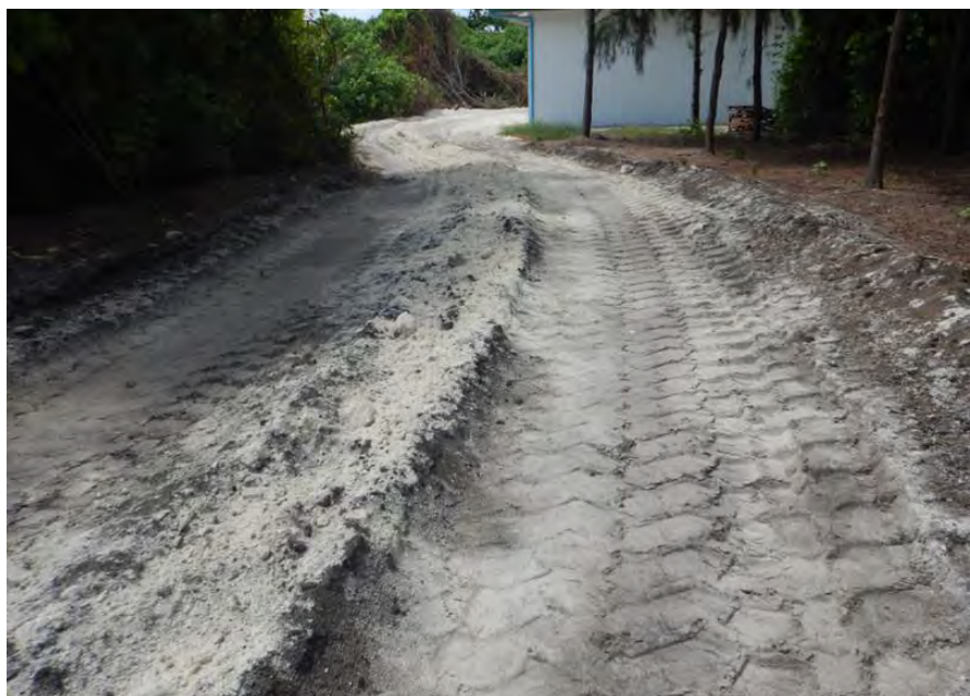
Figure 16: Impact on roads from heavy vehicle transport in an island in Maldives
