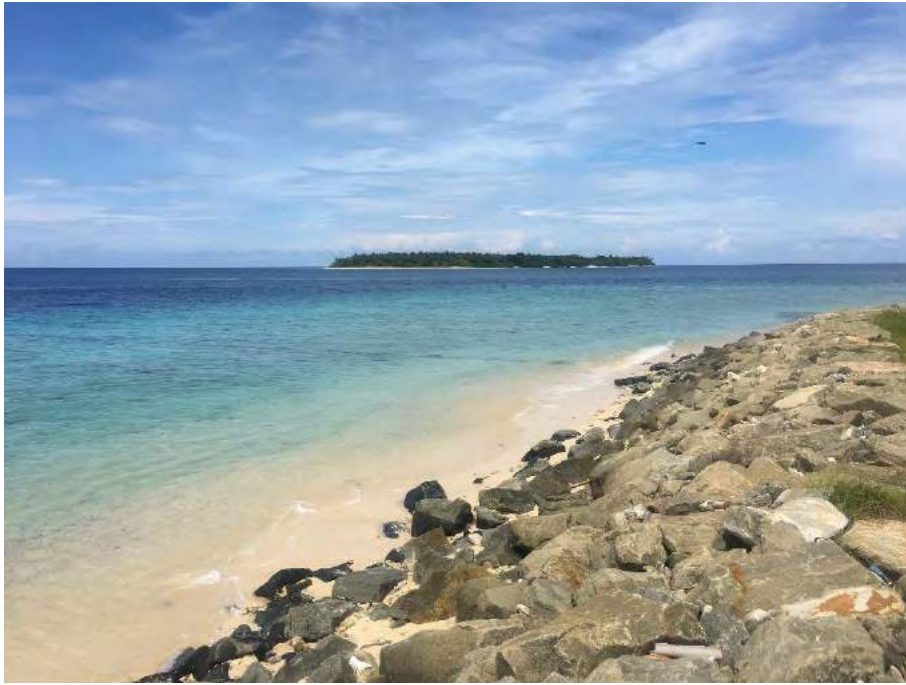
Figure 12 Shoreline adjacent to IWMC being protected by rock boulder revetment
