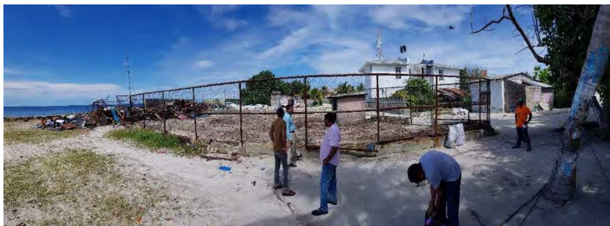
Figure 9 Panoramic view of the existing IWMC
