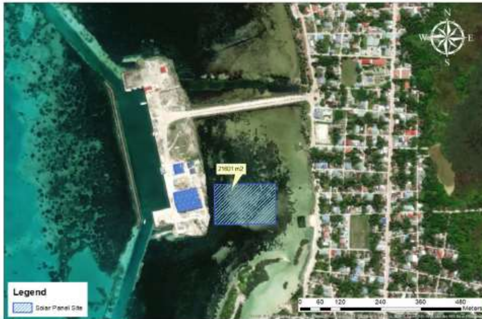
Figure 13 HulhudhooMeedhoo Floating Solar Site
