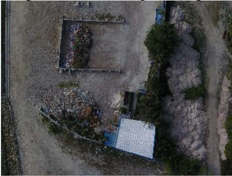
Figure 4: Aerial view of the existing IWMC at Villingilli 23
