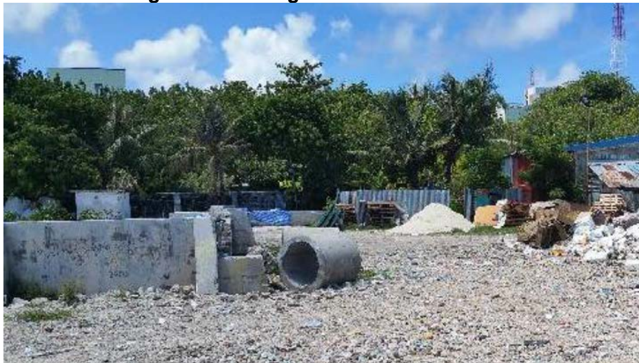
Figure 5: Existing condition of the IWMC
