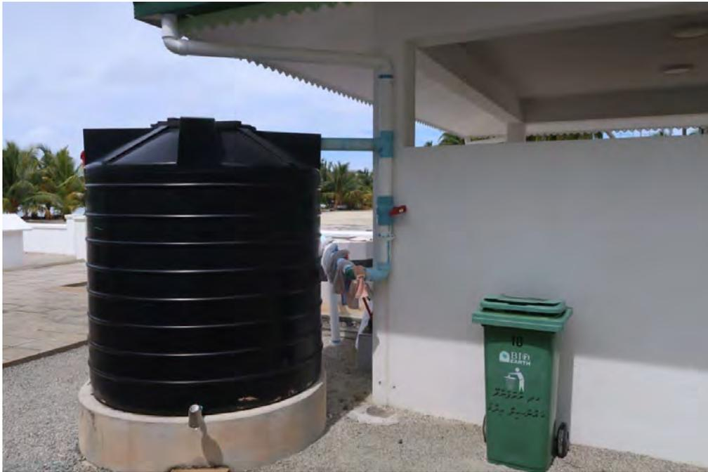
*Figure 1.3: A simple Rainwater Harvesting setup in a mosque in GDh. Rathafandhoo (The most common method of Rainwater Harvesting system in islands) (Source: Authors)*
