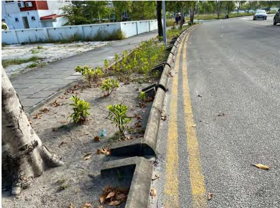
*Figure 2.12: In almost every street in Hulhumale', stormwater is managed entirely by infiltration drainage facilities without using a piped drainage system. (Source: Authors)*
