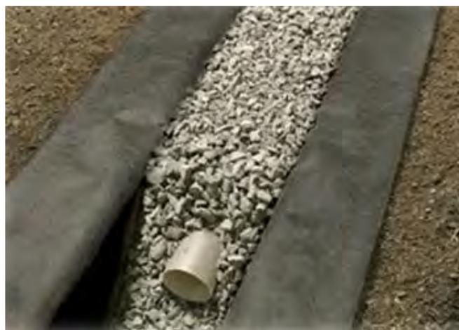
Figure 1.9: A filter drain under construction (Source: [edensstructural.com](http://edensstructural.com))
