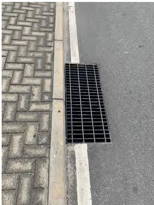
*Figure 2.5: Grating of a road drain inlet installed in the ring road of the capital city Male' (Source: Authors)*
