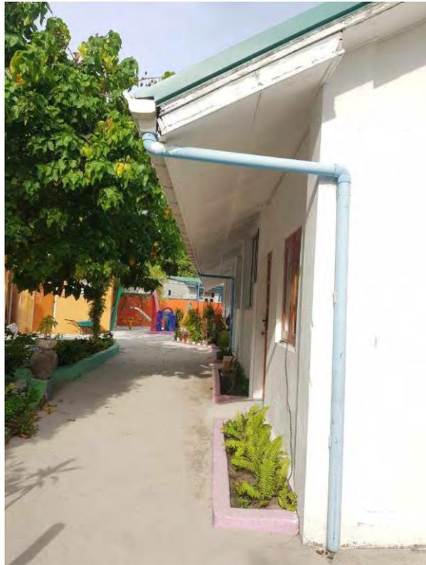
*Figure 8: A downpipe connected to the roof gutter has been left to discharge rainwater directly to the ground surface (a common practice in the islands) (Source: Authors)*
