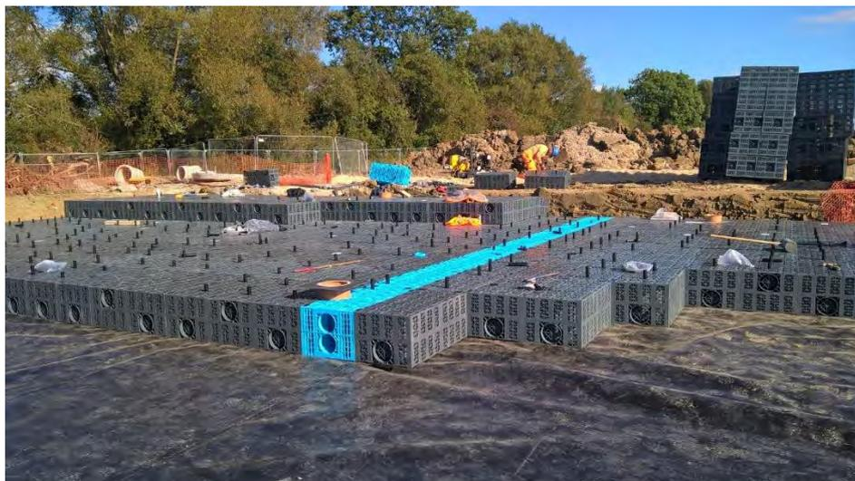
Figure 2.25: Geocellular tank units are being installed in a park (Source: [blog.wavin.co.uk](http://blog.wavin.co.uk))
