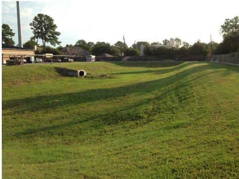
*Figure 1.12: Example of a large infiltration basin suitable for areas with plenty of open free space
