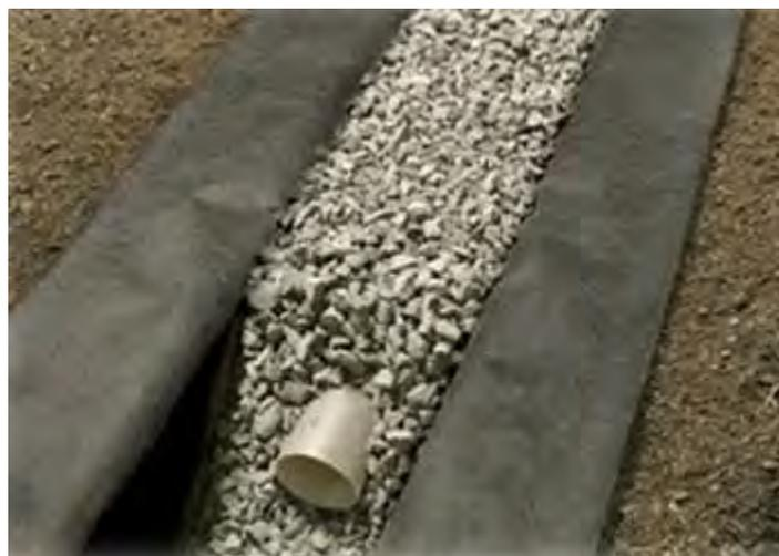
Figure 2.22: A filter drain under construction (Source: edensstructural.com)
